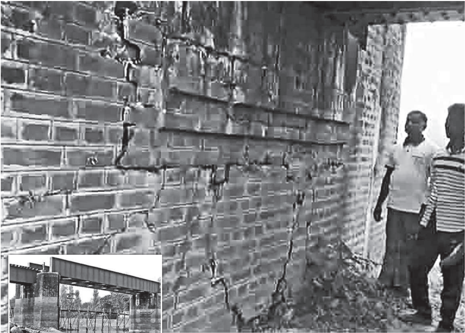
Railway workers take a look at the cracks that developed in one of the piers of the century-old Bheramara rail bridge, inset , over the Ghaghot river near Gaibandha rail station. The photo was taken recently.
