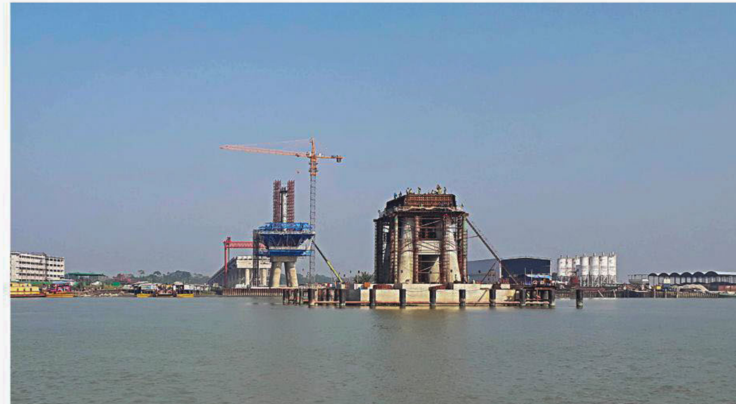
Construction work of Payra Bridge in Lebukhali area of Patuakhali is still incomplete although the scheduled completion date was April this year.
