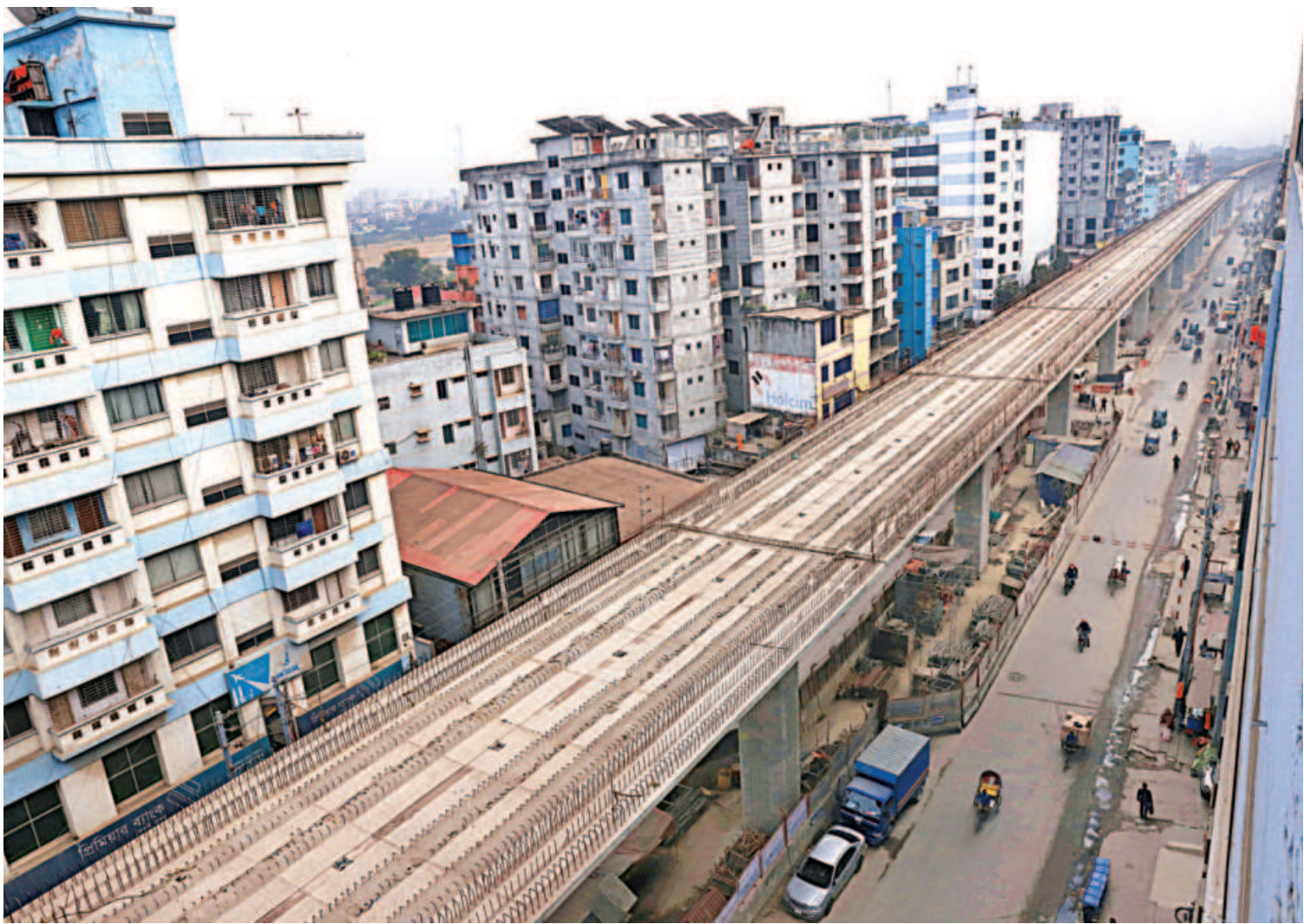
A portion of the metro rail's viaduct in Shewrapara in the capital. The project authorities are set to start installing rail lines on the elevated structure on January 1. The photo was taken yesterday.
