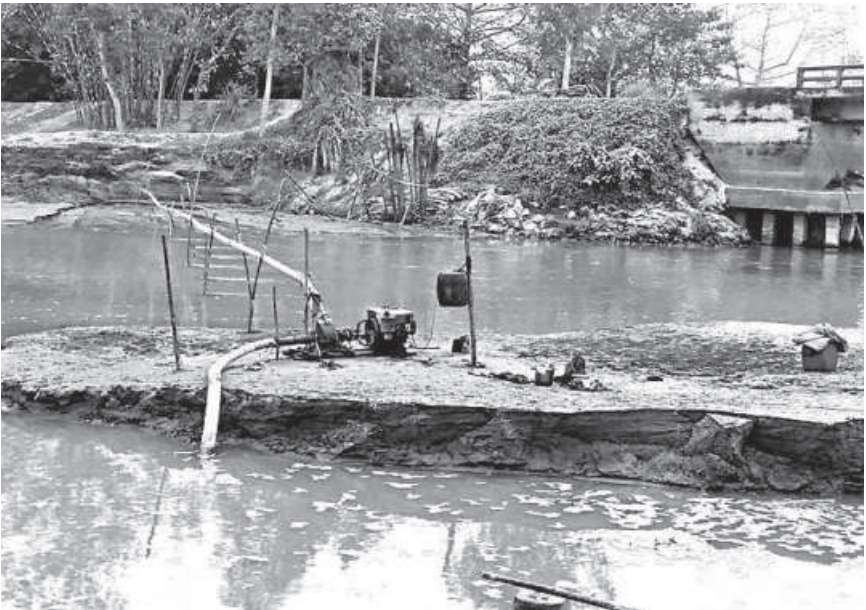
An irrigation pump has been set instead of using dredger for river excavation, posing erosion threat to the nearby bridge, road and homesteads in Gaibandha’s Sundarganj upazila.
