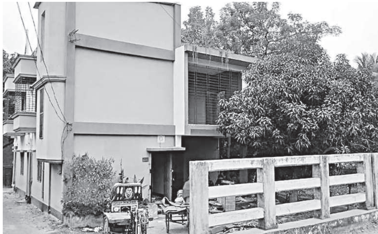
Occupier of a house, built apparently on the land of the Ichamati river at Kadomtali in Pabna town, shift belongings from the structure yesterday as the district administration is going to start a drive to demolish illegal structures from the river areas in the district headquarters today.
