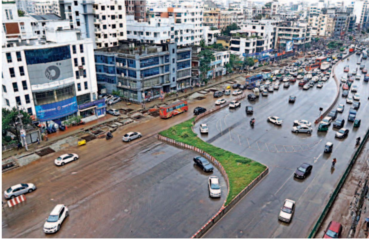
This U-loop on Airport Road near Uttara-3 was opened to traffic around six months back, with an aim to ease traffic congestion.
