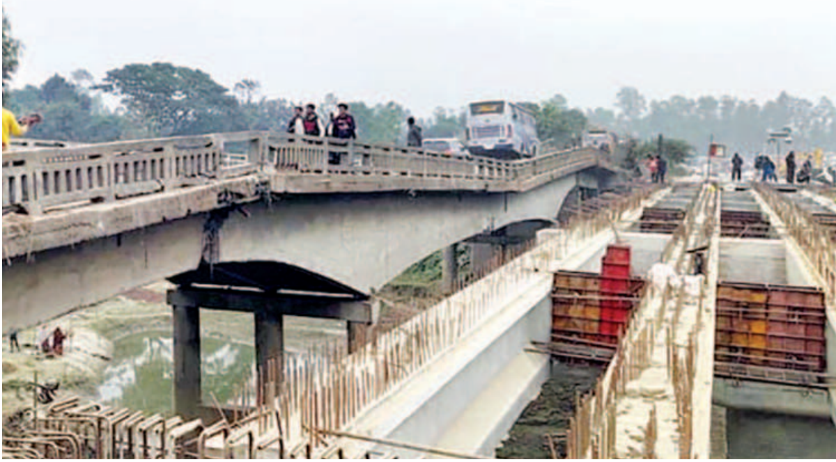
A part of this 80-metre bridge in Vuiagaati area of Sirajganj’s Raiganj upazila subsided on Wednesday night, disrupting traffic movement on the Hatikumrul-Bogura highway. Construction of an alternative bridge, just beside the dilapidated one, has not ended in a year.
