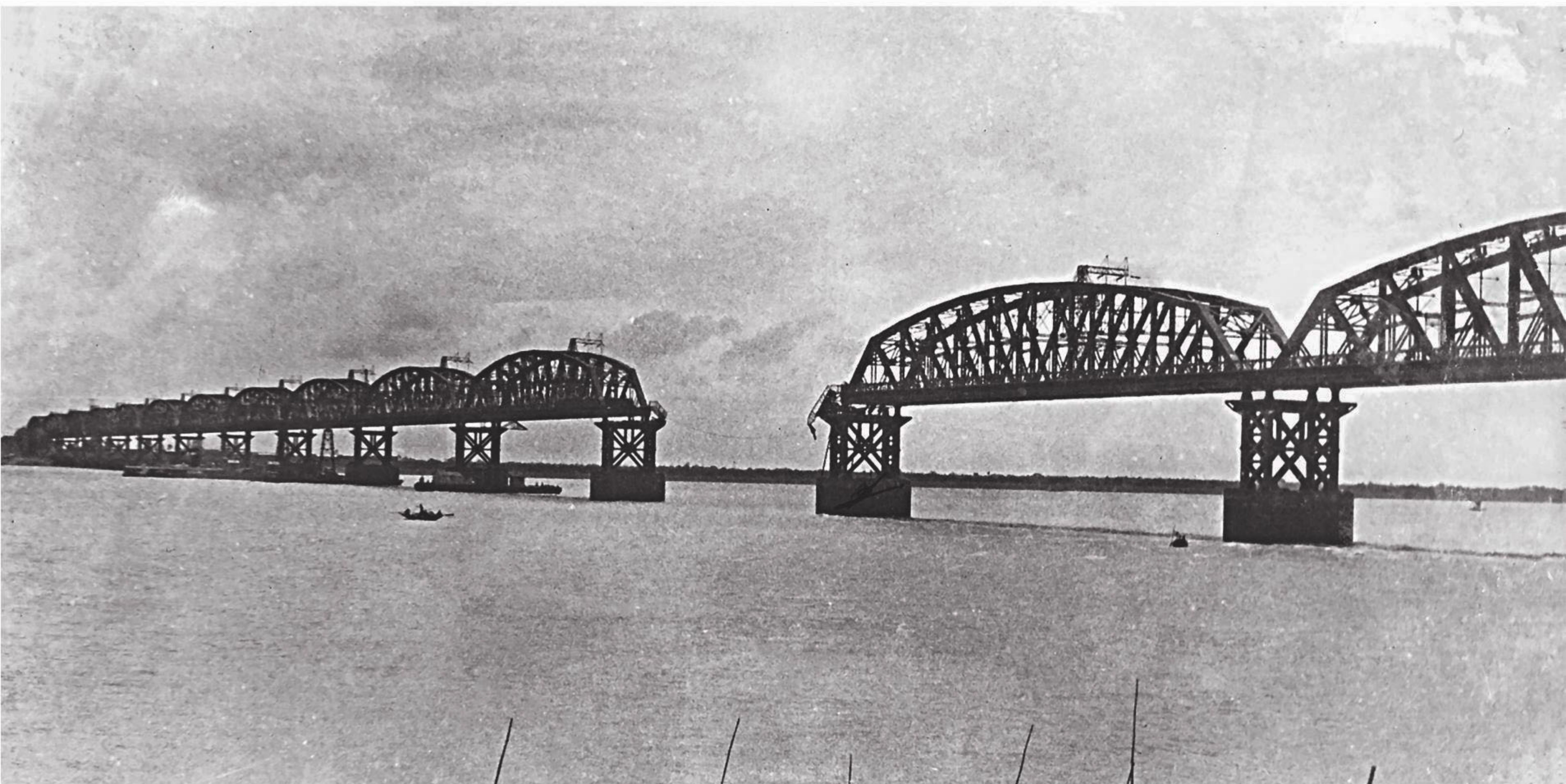
A partially damaged Hardinge Bridge, 1971.
