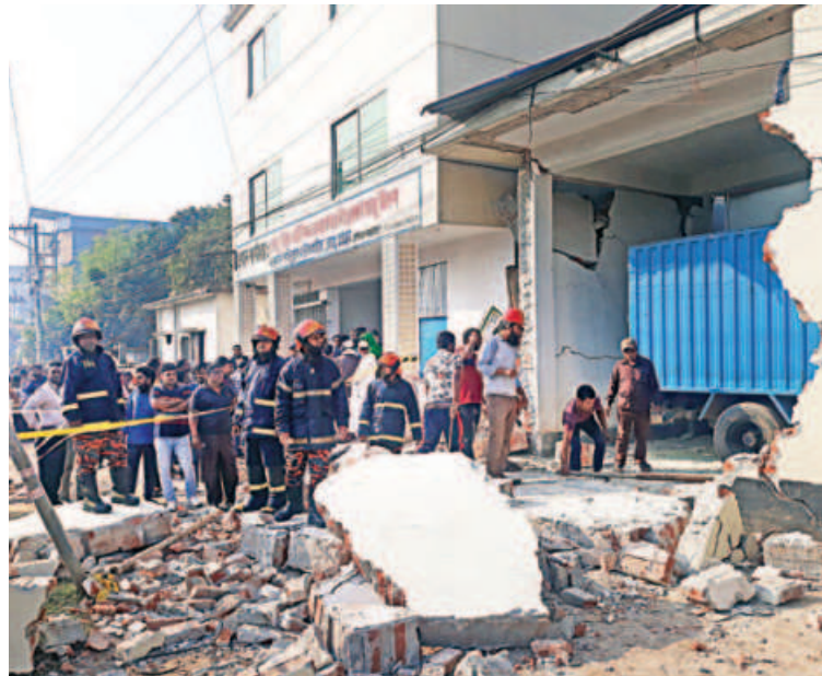
An explosion destroyed the walls of a sweater factory in Ashulia, killing a woman and injuring five people. PHOTO: COLLECTED
