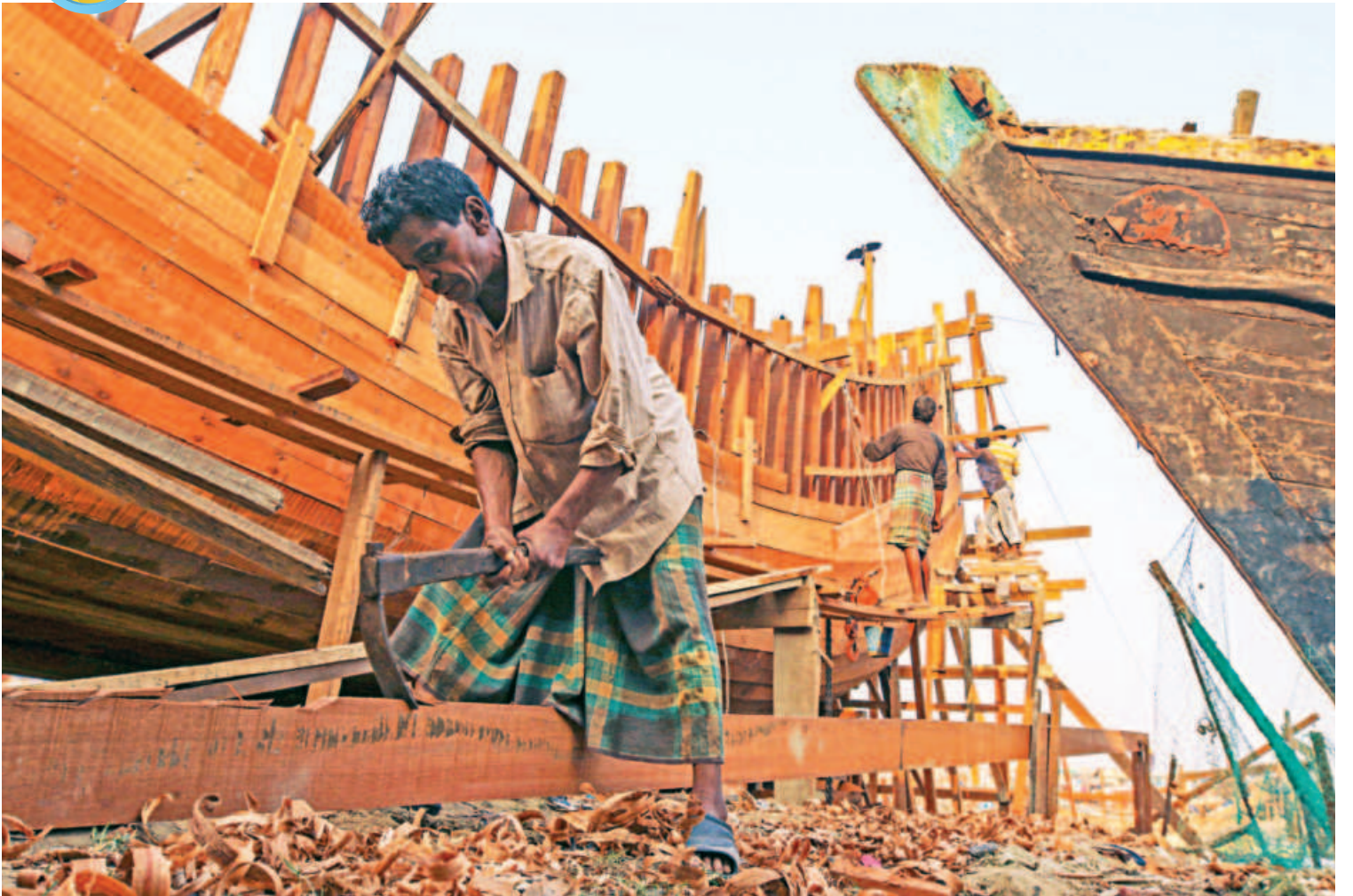
With rows of nearly finished and some unfinished wooden boats lined up by the banks of Karnaphuli and craftsmen busy working, Fisheryghat area in port city is abuzz with activities these days. Each of these watercrafts requires rigorous craftsmanship for around three months. The vessels then set sail on the Bay of Bengal for fishing. According to boat makers, the dry season is the ideal time for making fishing boats, which come with a price tag as high as Tk 1 crore.
