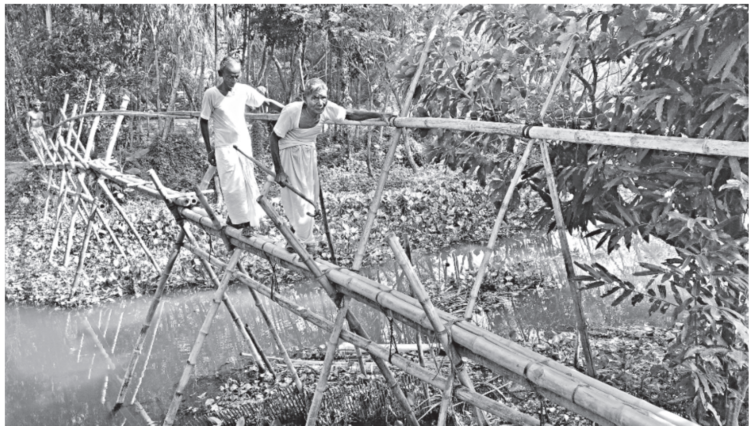
Two elderly men cross the bamboo bridge over the canal amid risk of accident in Gopalganj's Kotalipara upazila.
