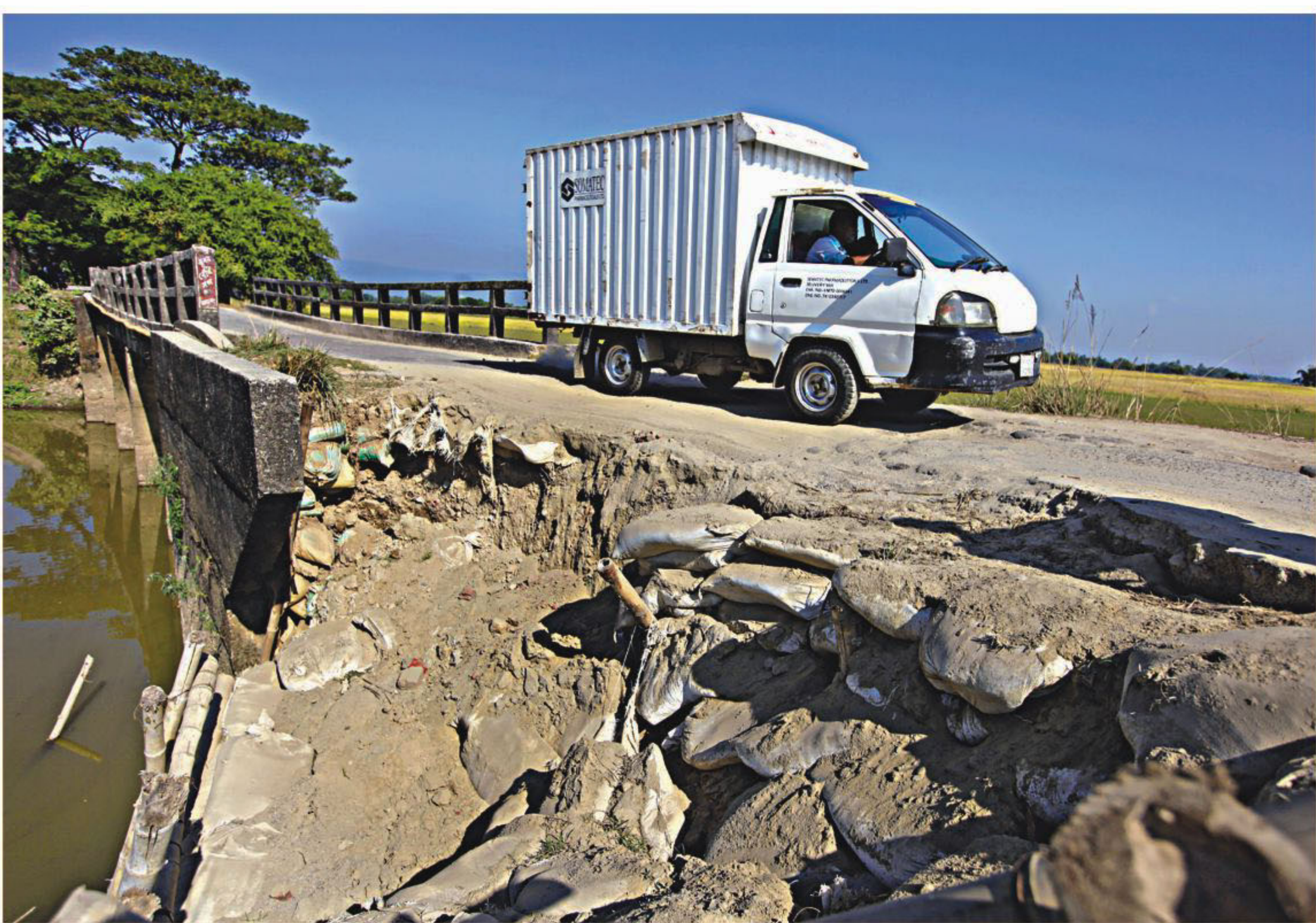
A van crosses a badly damaged bridge in Paschim Jaflong Chotkhal area in Sylhet's Gowainghat upazila yesterday. Locals said part of the bridge's approach road caved in six months ago, after which the LGRD did some makeshift repairs using sandbags and bamboos. Those too were flooded away by recent rains.
