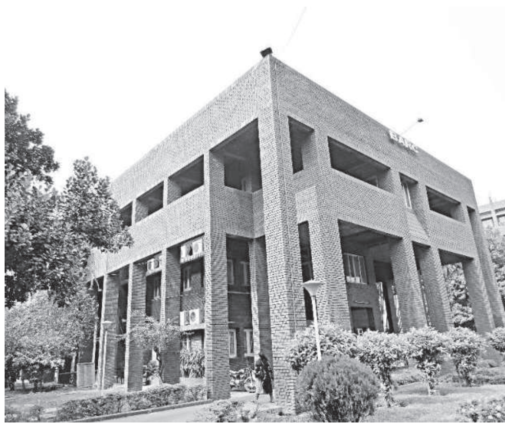
It is difficult to miss the 'poetics' of brick in the conceptualisation and organisation of the BARC headquarters building.
