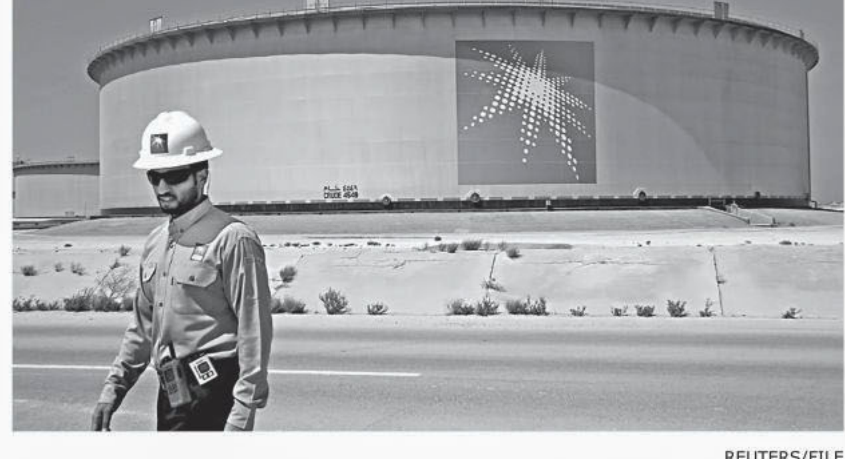
An Aramco employee walks near an oil tank at Saudi Aramco's Ras Tanura oil refinery and oil terminal in Saudi Arabia.
