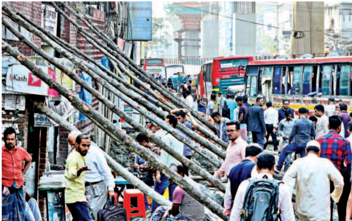
Pedestrians traverse around and under logs that are precariously supporting an unstable building wall. This whole situation is a result of authorities digging up the road for sewage line work. This photo was taken on Tuesday near Dainik Bangla intersection.
