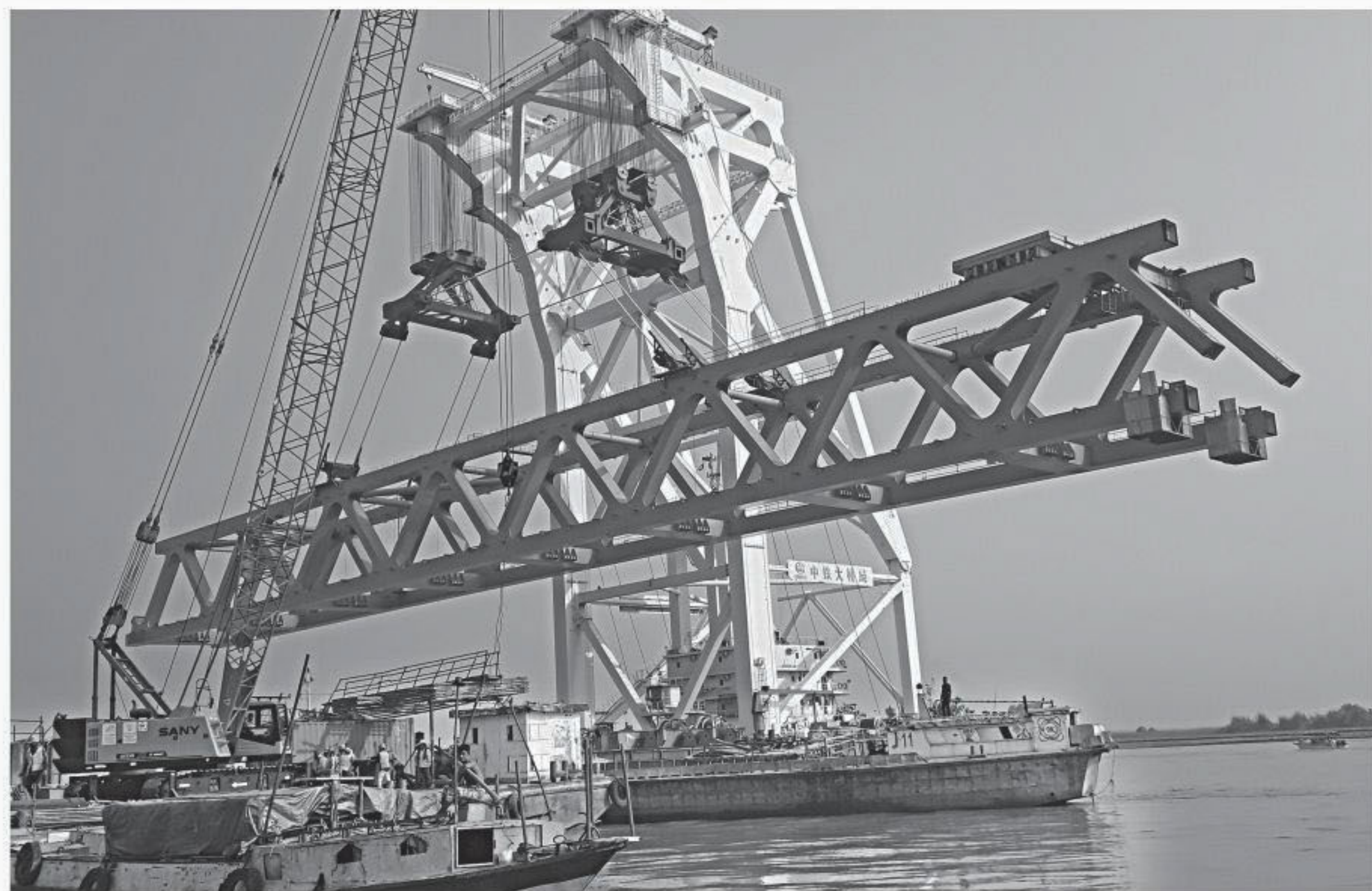
The 17th span of the under-construction Padma Bridge is being taken near 22th and 23rd pillars yesterday for installation.
