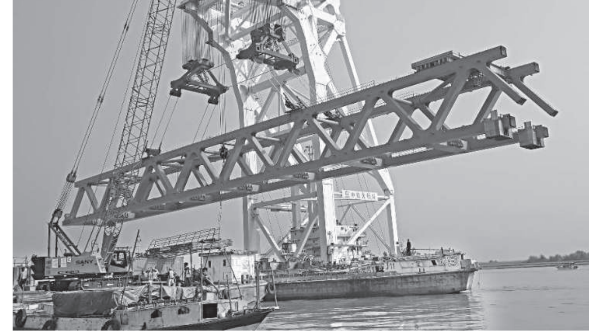
The 17th span of the under-construction Padma Bridge is being taken near 22th and 23rd pillars yesterday for installation.
