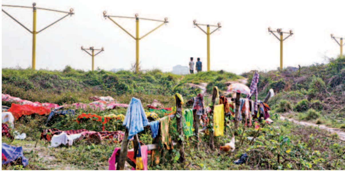
Two youths stand beside a marker beacon, hoping to see a plane fly by. This area, known as Middle Marker, is a restricted zone that provides directions to planes for safe landing on runway. Due to damaged walls and lack of monitoring, it has become a recreational spot for locals. They also dry clothes and use a part of the airport land for farming. The photo was taken yesterday afternoon.
