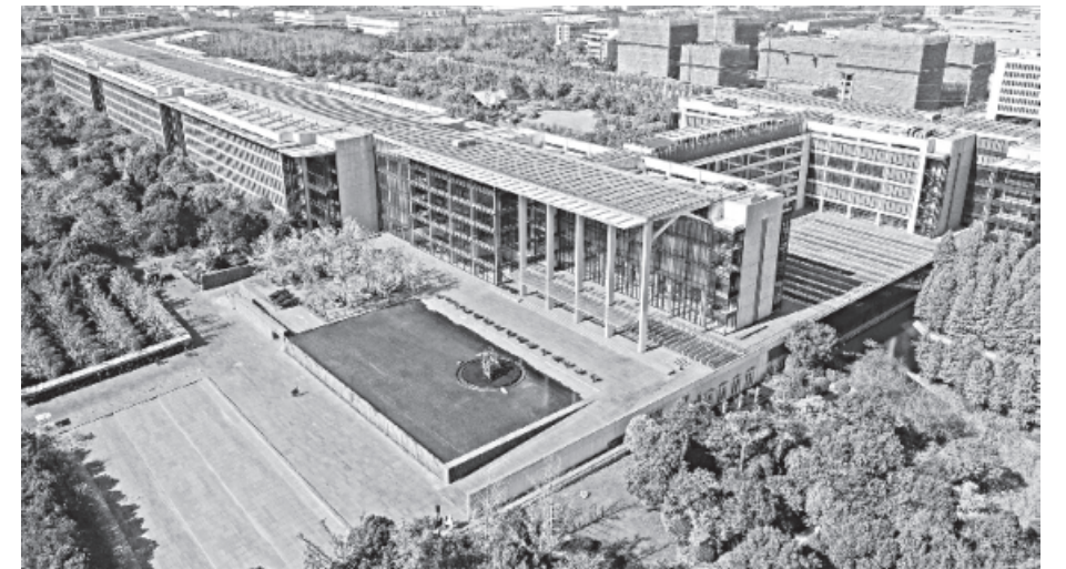
This aerial photo shows a building at the Huawei research and development centre in Shanghai on November 19.
