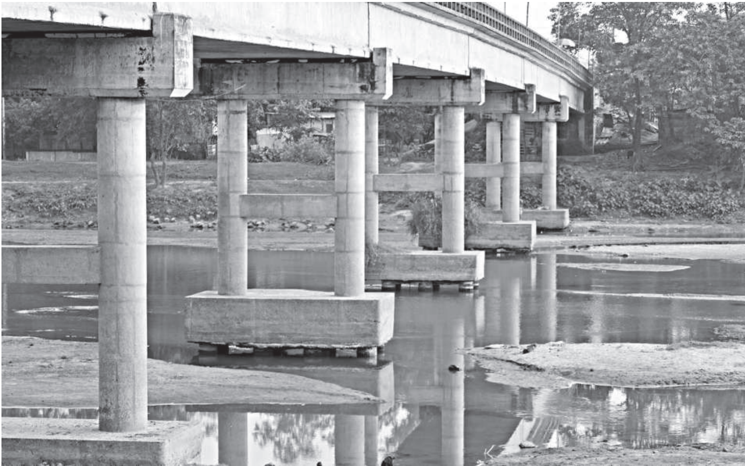
Due to mindless sand lifting in close proximity of Majadanga Bridge in Dinajpur Sadar upazila sediments around the piers have already been washed away, making it vulnerable to collapse.
