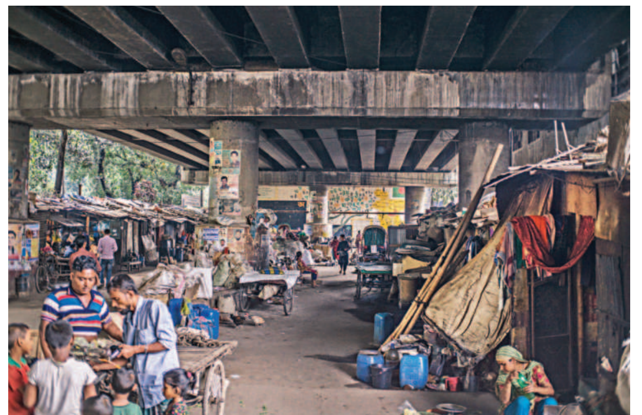
A lion's share of the road underneath the Bijoy Sarani-Tejgaon flyover has been taken over by low-income people, who have set up shops and shanties, keep their rickshaw vans parked here, and even rear chicken. As a result, vehicular movement on the road has become constricted. The photo was taken yesterday. PHOTO: RASHED SHUMON
