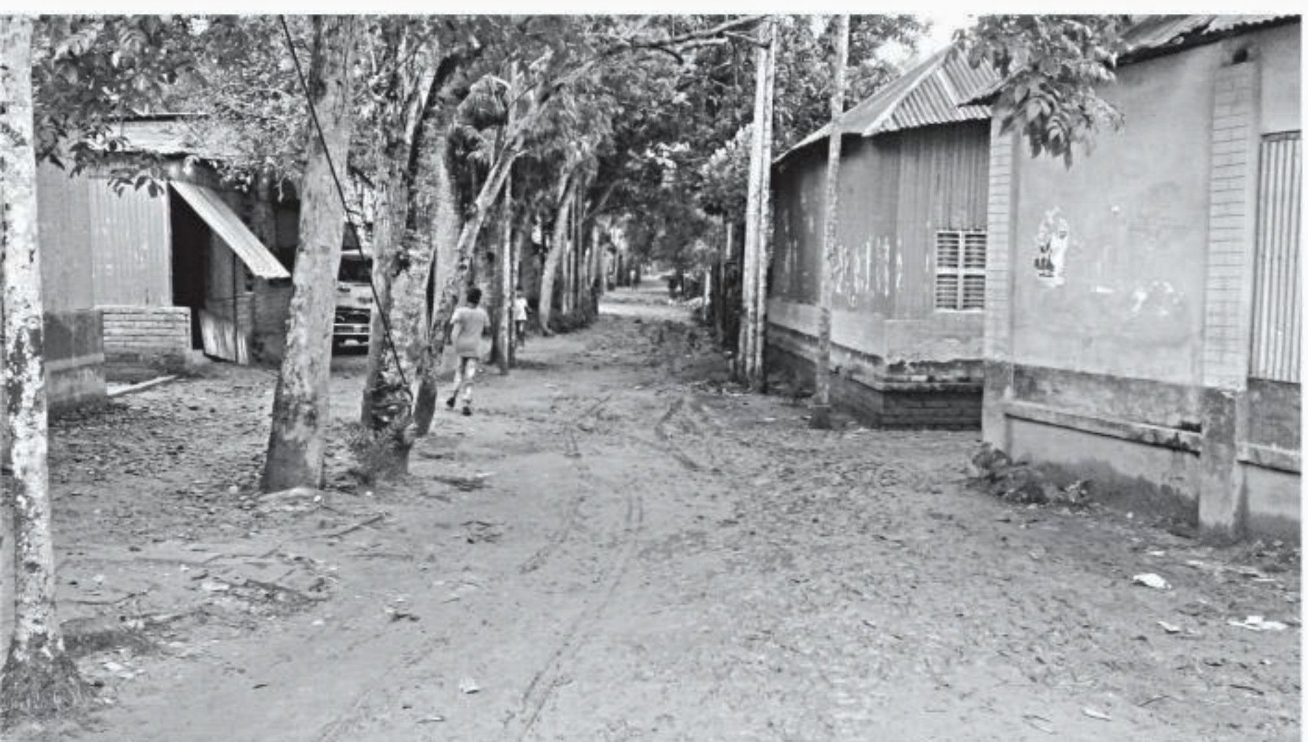
During the rainy season this two-kilometre-long muddy road in Faridpur's Madhukhali upazila remains virtually unusable for vehicles.
