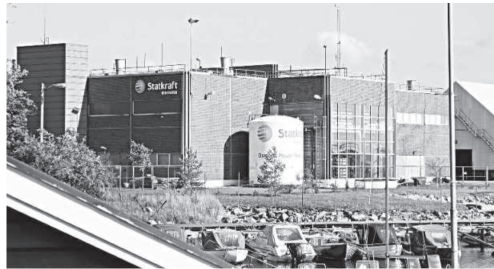
Statkraft osmotic power prototype is the world's first osmotic power plant.
