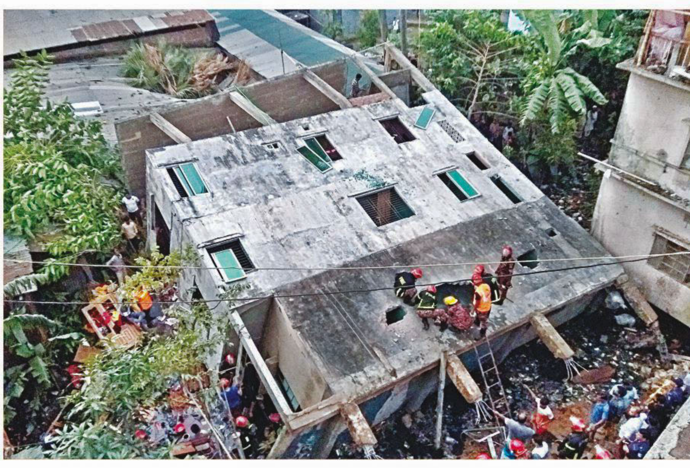
Firefighters look for survivors after a three-storey building tilted to its side and collapsed in Narayanganj city's Baburail area yesterday. A 10-year old boy was killed and five others were injured when the building collapsed on a canal, possibly due to faulty piling.
