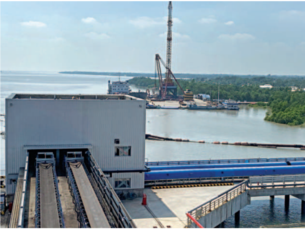
The main structure of the coal-fired Payra Power Plant in Patuakhali's Kalapara upazila. Right , the jetty of the plant will be used to unload coal from vessels. The coal will be carried along on conveyor belts to the coal storage silo. The photos were taken on Tuesday.
