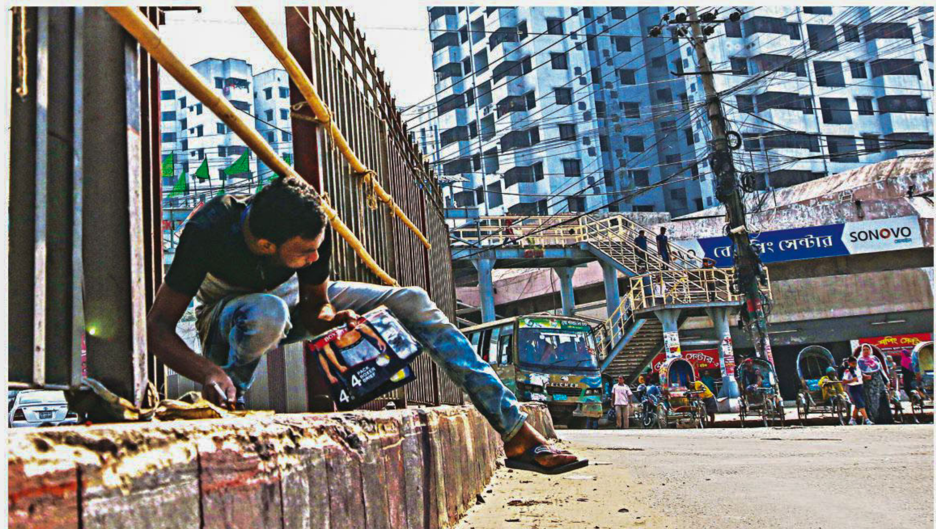
Two bamboos placed perpendicularly to prevent pedestrians from jaywalking through this gap in a road divider barricade cannot deter a youth from stooping and squeezing through. There are three foot-overbridges in the vicinity, one of which can be seen in the photo. The photo was taken from Chattogram city's EPZ intersection yesterday.
