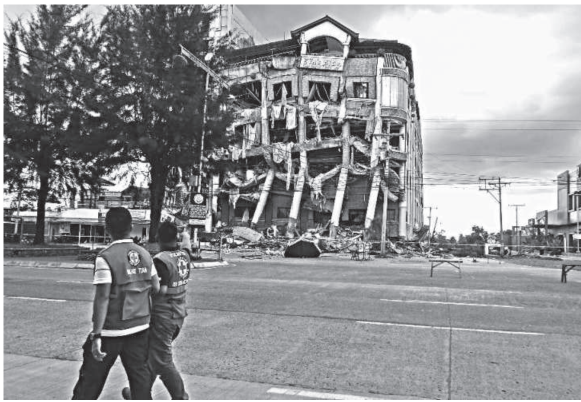
Local Red cross personnel walk past a damaged building after a 6.5-magnitude earthquake hit Kidapawan town, north Cotabato province, on the southern island of Mindanao, Philippines yesterday. At least five people were killed and nine people were injured in the earthquake.
