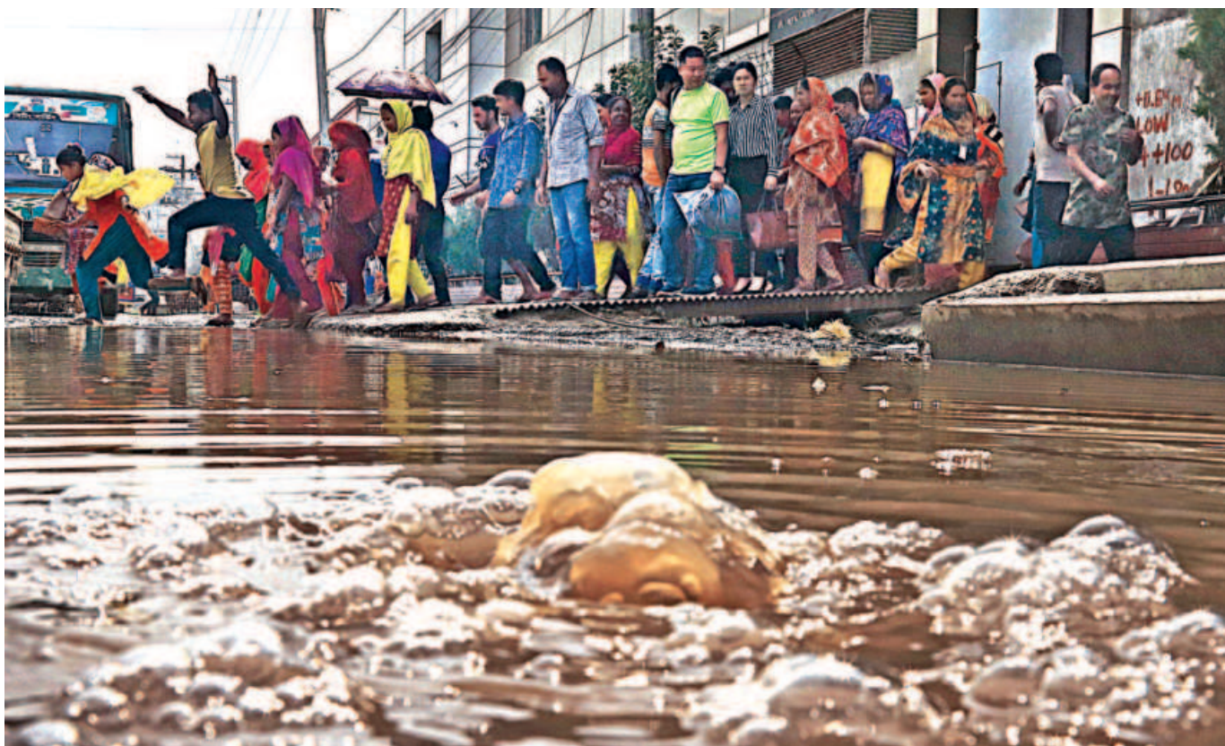
Pedestrians leaping over mud and water accumulated on roads is a common occurrence. Bubbling water, however, is not. Authorities had dug up this road, and in the process damaged a gas line underneath. The road was later patched up, but not the pipeline, said locals. Besides gas fuel being wasted, this could also turn into a fire hazard when the water recedes. The photo was taken on Tuesday from Maleker Bari area in Gazipur.
