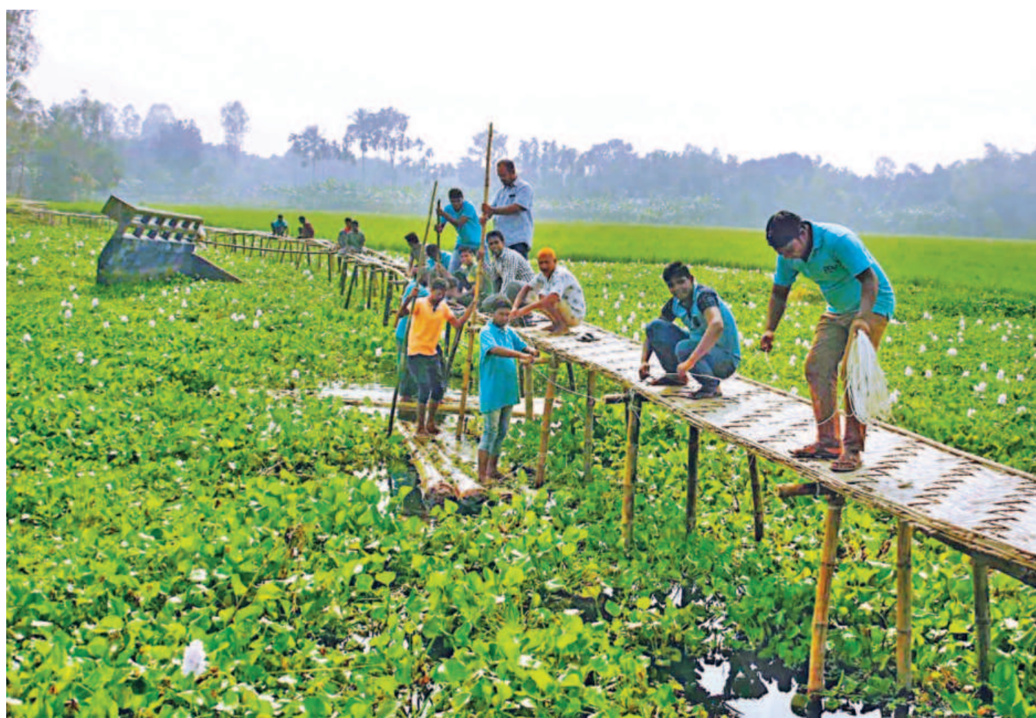
Locals building a bridge with bamboo on a canal in Gaddimari village of Lalmonirhat's Hatibandha upazila. They are putting in the effort after failing to get any help from the authorities to repair a bridge that collapsed in 2015. The photo was taken on Friday.
