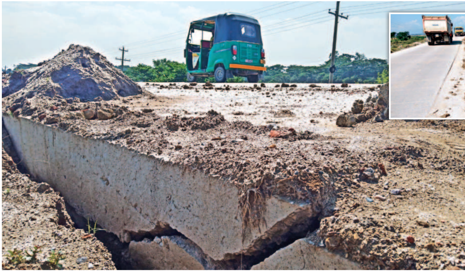
This Tk 700 crore project to construct a highway from Sylhet to Companyganj uses Reinforced Cement Concrete (RCC), for the first time in Bangladesh. Work hasn't finished yet, but cracks have already appeared on the road. The construction company attempted to cover the cracks with dirt near Sylhet Hi-tech Park, according to locals. The photos were taken on Monday.
