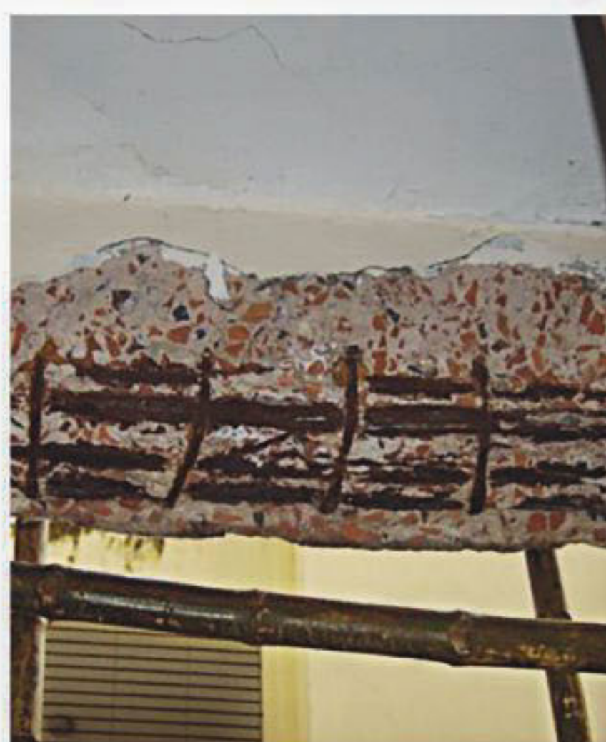
Deterioration of concrete due to corrosion of steel in concrete (Top – Slab, Bottom Left – Column, Bottom Right – Beam).
