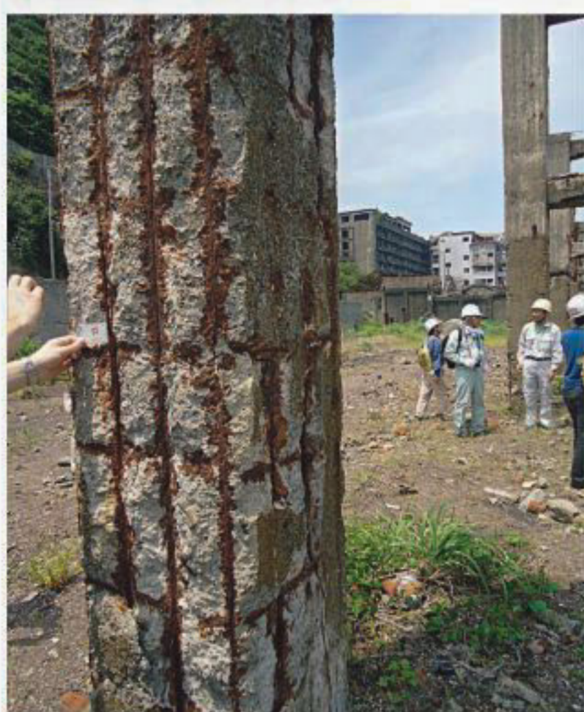
Deterioration of concrete due to corrosion of steel in concrete (Top – Slab, Bottom Left – Column, Bottom Right – Beam).
