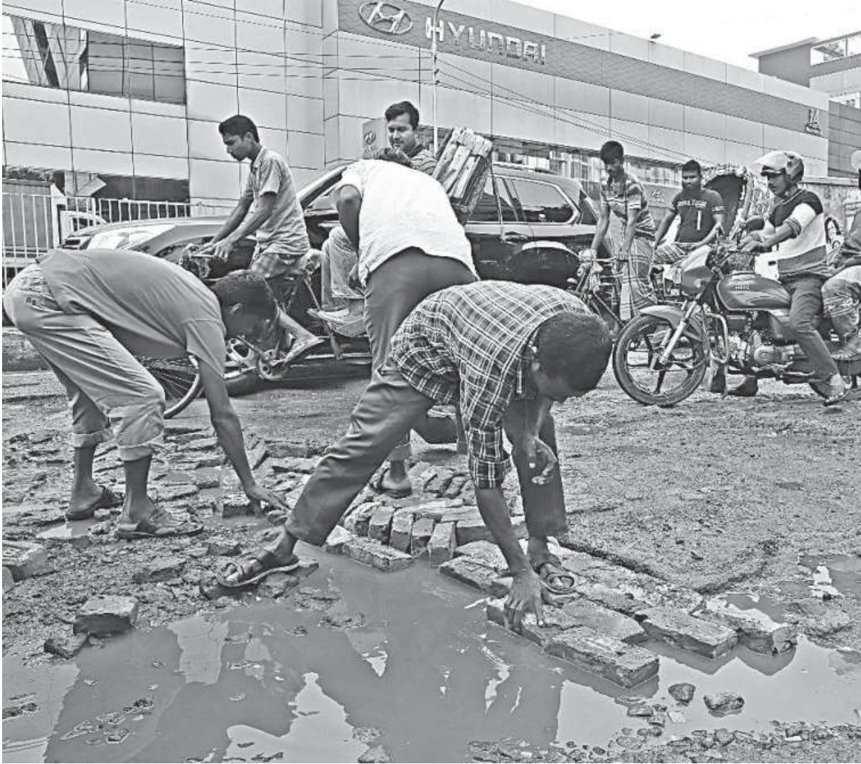
City corporation workers put bricks over a pothole on Gulshan-Link Road as this part of the road has been in a bad shape for a while. They also sprinkled some sand on top, and satisfied with the patch-up work, left. Meanwhile with potholes and muddy surface, travelling on the road has become quite risky. The photo was taken yesterday.
