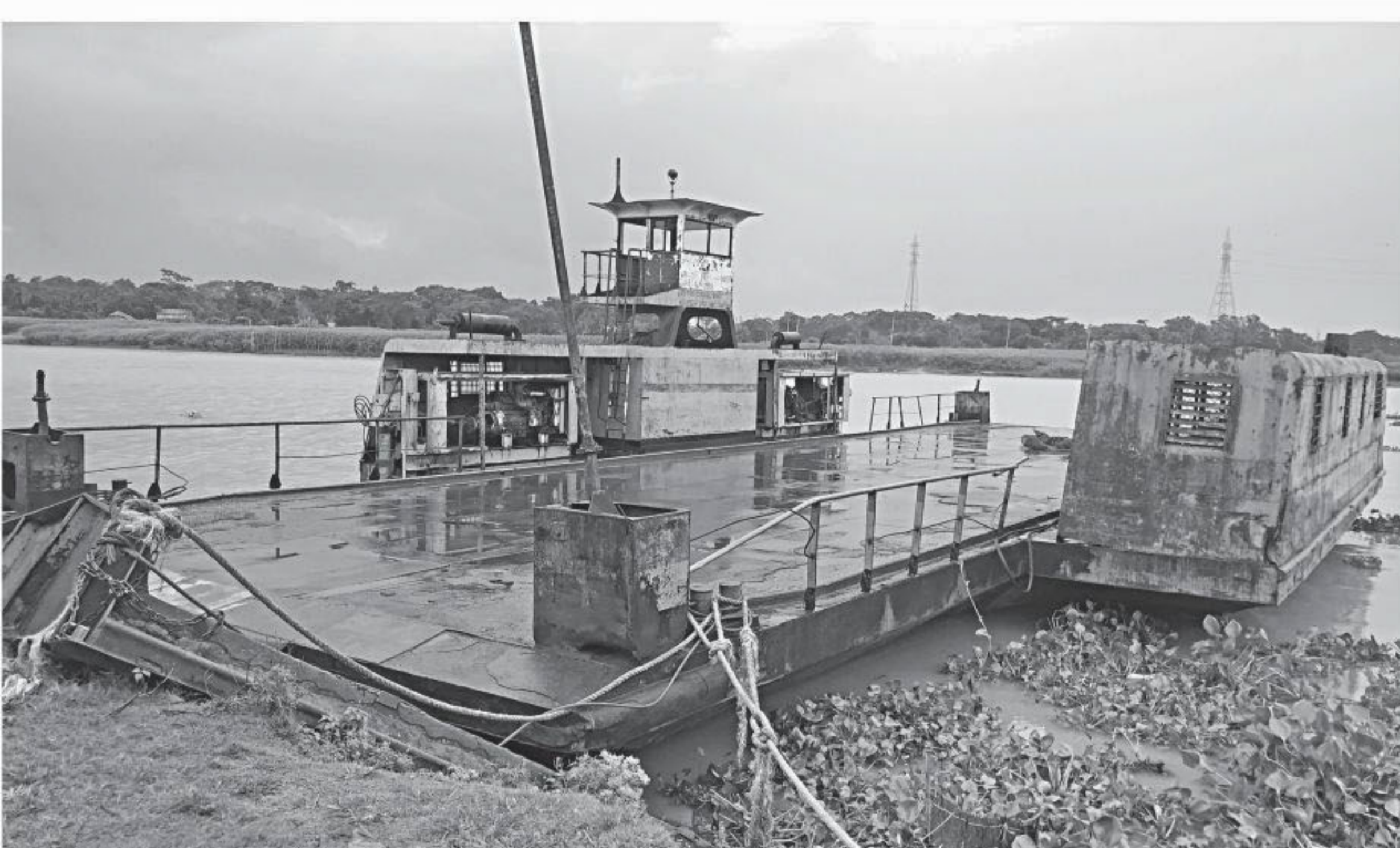
This ferry at Kazirtak terminal in Madaripur Sadar upazila is decaying as it has remained unused since a bridge was built on the Arial Kha river over four years ago. Three pontoons at the terminal are also rotting due to the same reason, thanks to the callousness of the authorities concerned.
