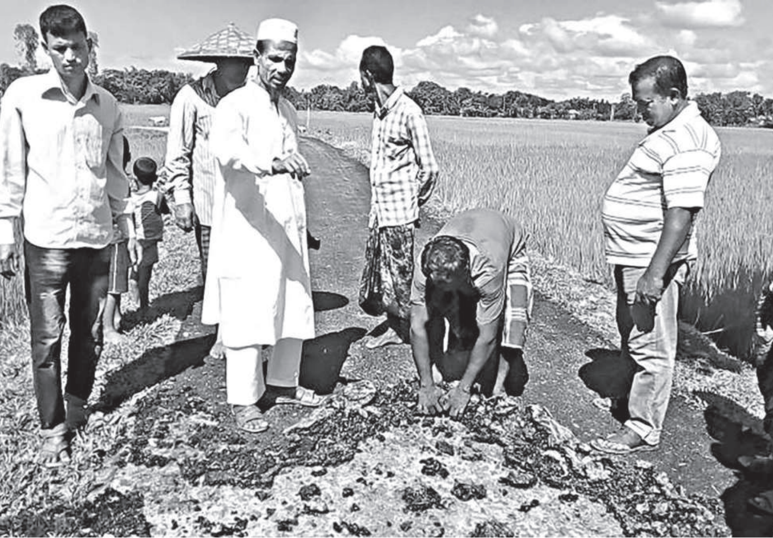
The newly completed carpeting of Bishnathpur-Gouripur road in Juri upazila of Moulvibazar gets removed with bare hands, bearing testimony to the low quality work. The photo was taken on Thursday.
