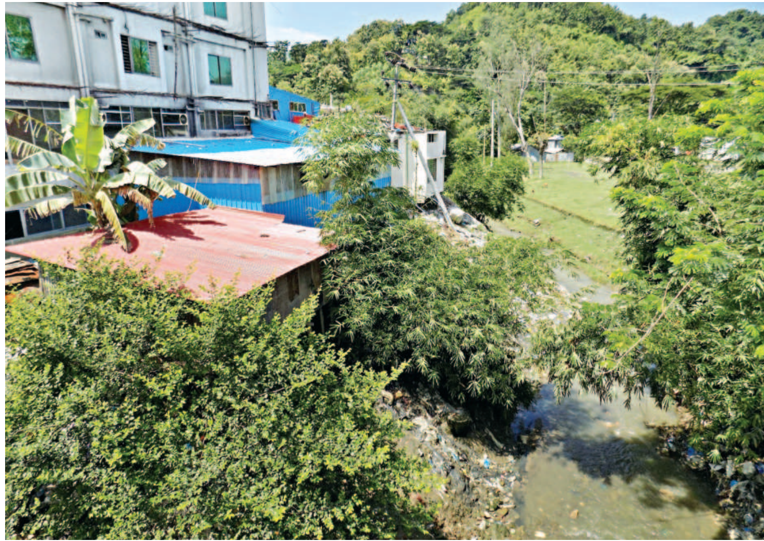
A chhara, which was quite wide not too long ago, is barely visible due to illegal encroachment and the administration's negligence in Bandarban. The photo was taken recently.
