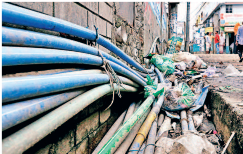
Wasa pipelines for supplying water to households have been set up through a sewage drain, with a possibility of raw sewage getting into the pipes, if leaked. Besides, the sewer is also blocked due to the pipes and garbage. The photo was taken from Muradpur area in Kadamtoli recently.
