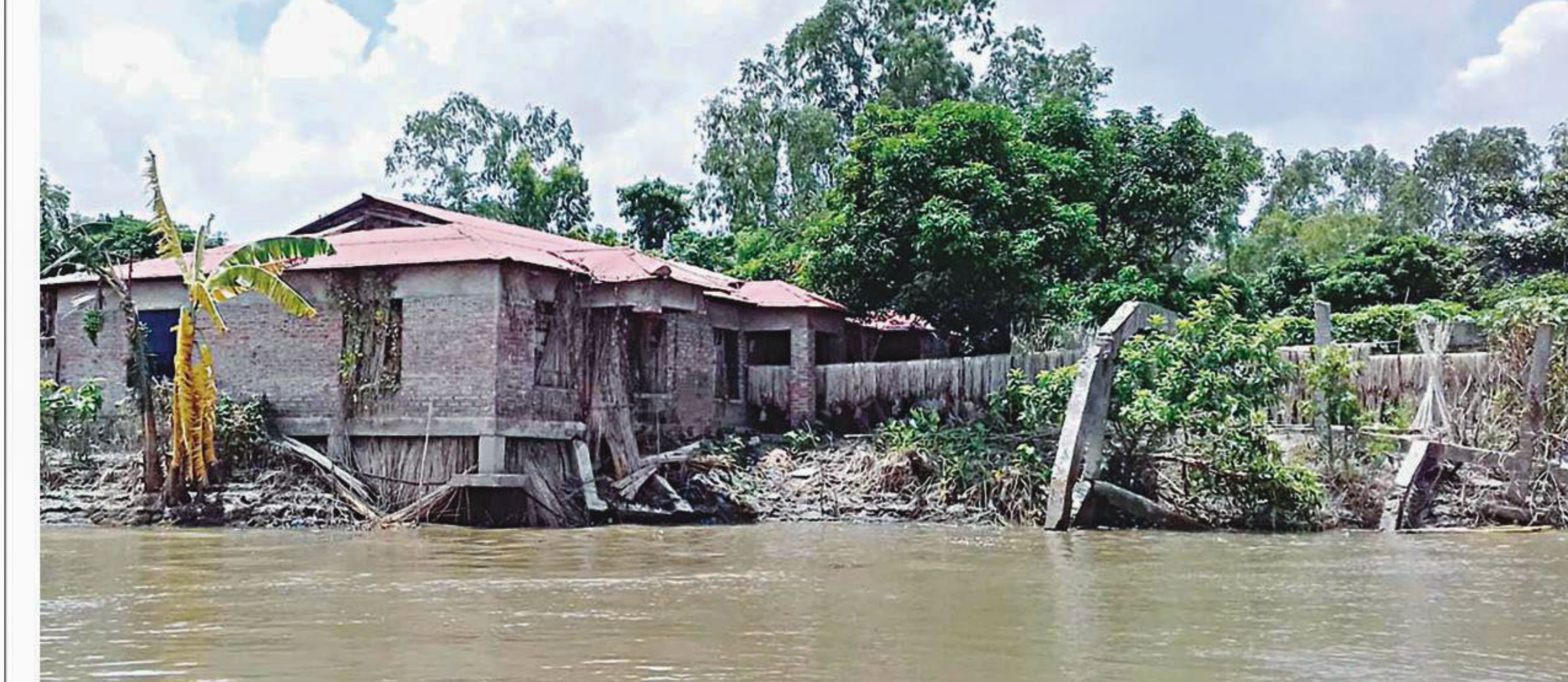
A shelter home in Bangla Bazar area of Gaibandha's Haripur union is in a sorry state in the absence of renovation. Built under a project named Ashrayan Prakalpa, the structure was hit hard by flood and erosion in 2015. The photo was taken recently.
