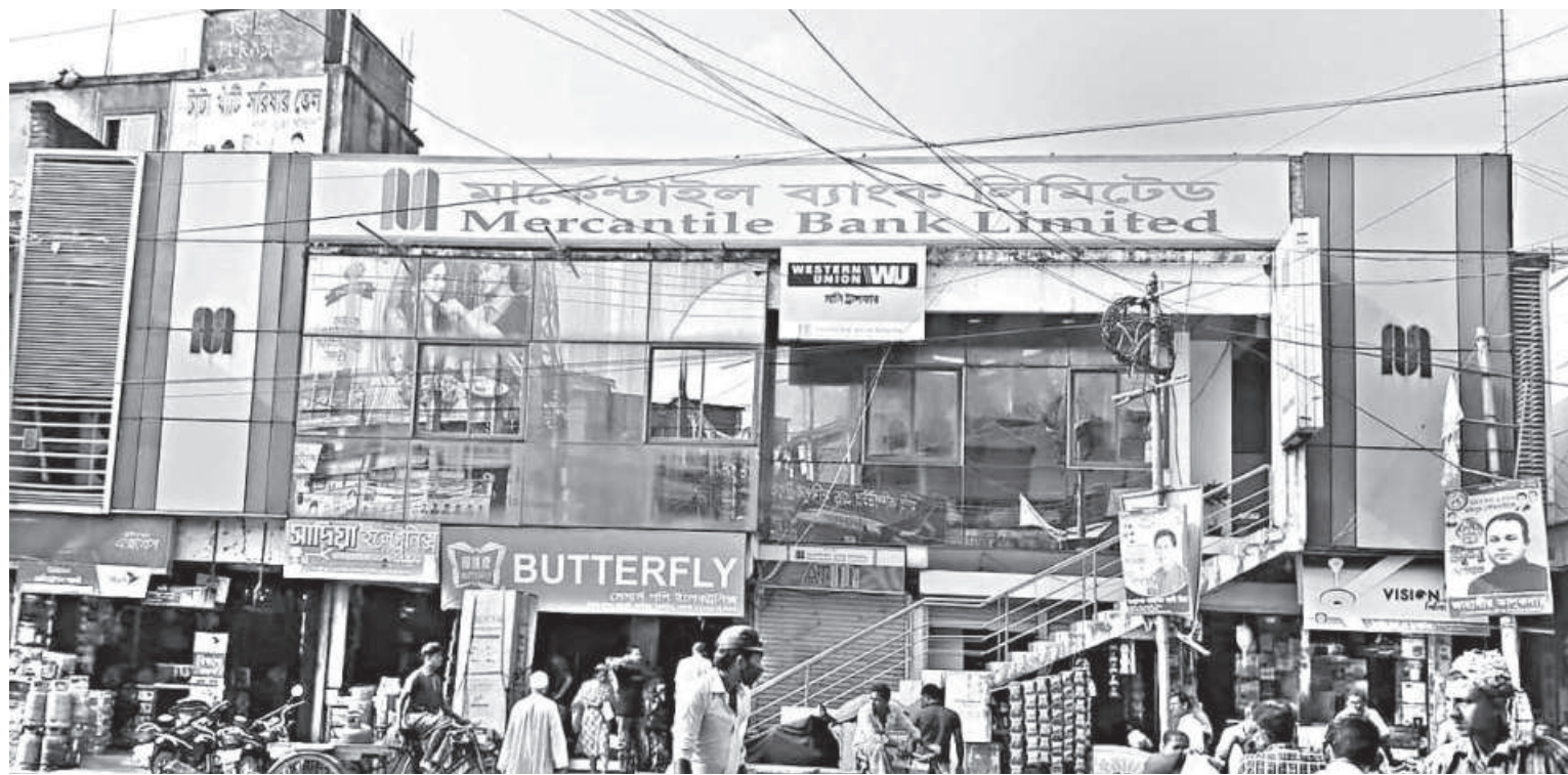
The district administration has served a notice, below, to the owners of this building at Mokhtar Foara Chattar under Sakhipur municipality area in Tangail, asking them to remove the structure as it was built allegedly on an illegally occupied government land.
