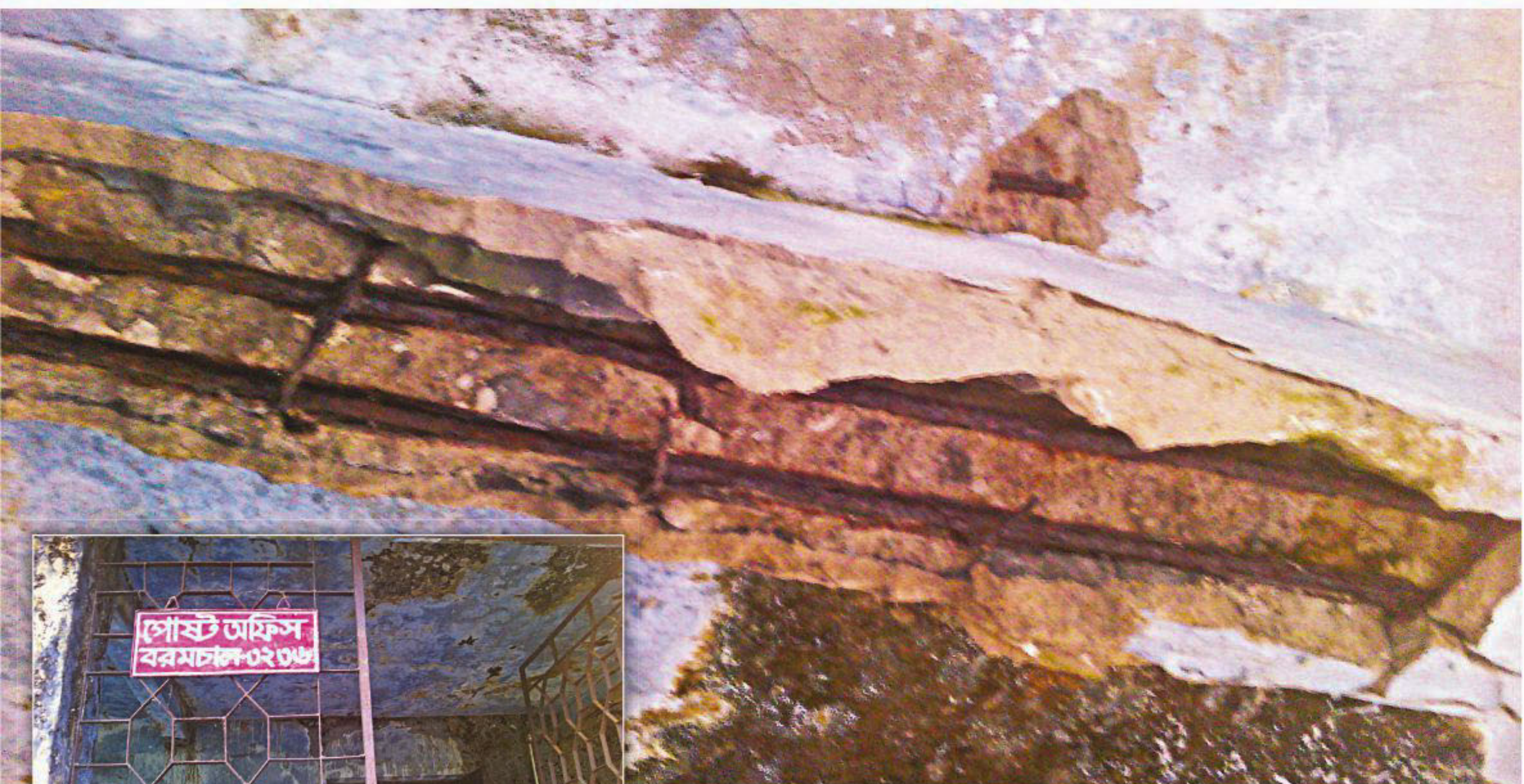
Exposed iron rods in a ceiling of a room inside the shabby building that houses Boromchal post office, inset, in Kulaura upazila.
