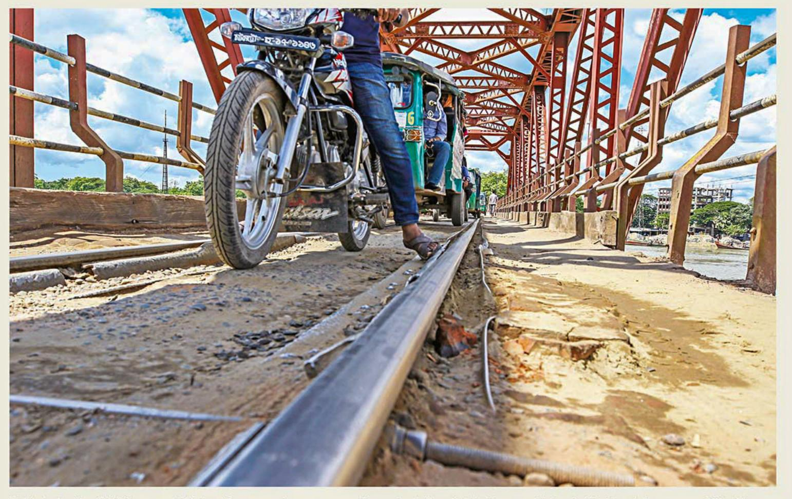
Built during the British era, a little less than a century ago over Karnaphuli river in Chattogram, Kalurghat Bridge is in a sorry state. The run-down bridge is now dotted with numerous potholes while its metal fencing and pedestrian decks have worn out in places, increasing the possibility of a serious accident any time. Long tailbacks have also become a common phenomenon there. Often times, the gridlock ensues way before entering the bridge. PHOTO: RAJIB RAIHAN
