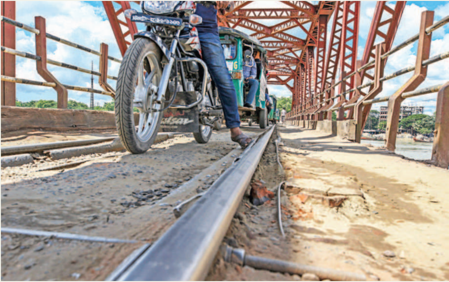
Built during the British era, a little less than a century ago over Karnaphuli river in Chattogram, Kalurghat Bridge is in a sorry state. The run-down bridge is now dotted with numerous potholes while its metal fencing and pedestrian decks have worn out in places, increasing the possibility of a serious accident any time. Long tailbacks have also become a common phenomenon there. Often times, the gridlock ensues way before entering the bridge.
