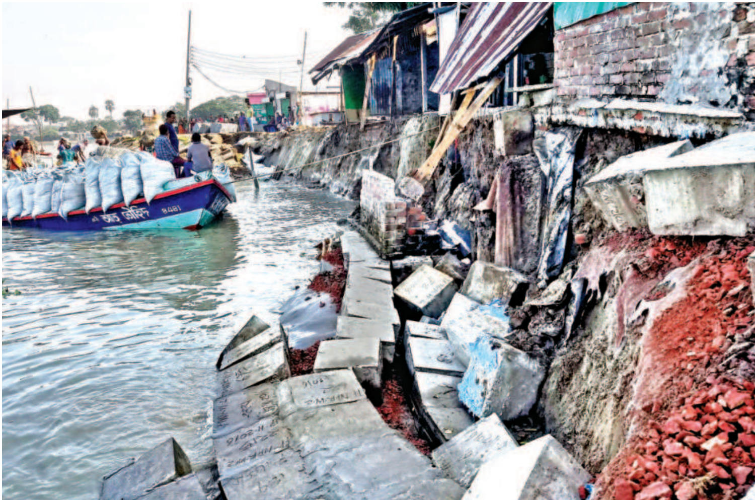
Part of the Chandpur town protection embankment goes into the Meghna in Puran Bazar Harisava area yesterday, a day after erosion hit the area. Water Development Board is dumping sandbags to check further damage to the embankment. The authorities said strong currents at the confluence of the Meghna and Dakatia rivers near the area were causing the erosion.
