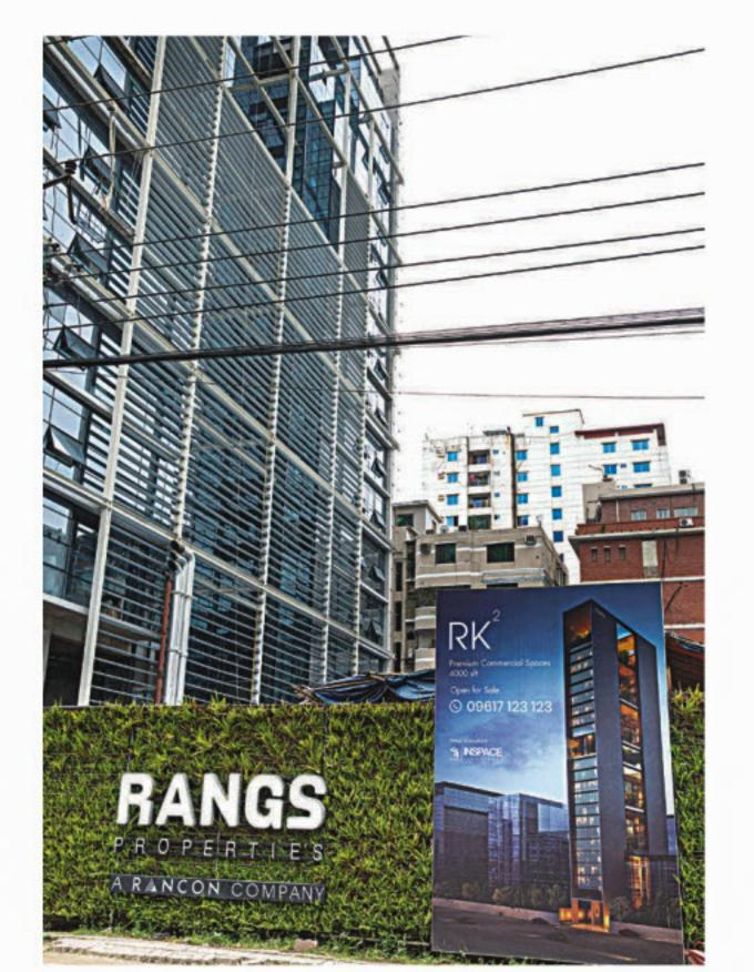
The new version features geotextile bags. These little bags or pockets work as a container for a compound mixture, where plants can grow. The fence is densely aligned with many of these bags making it a green fence. This version is sustainable and is 40 percent less expensive compared to the original version.
