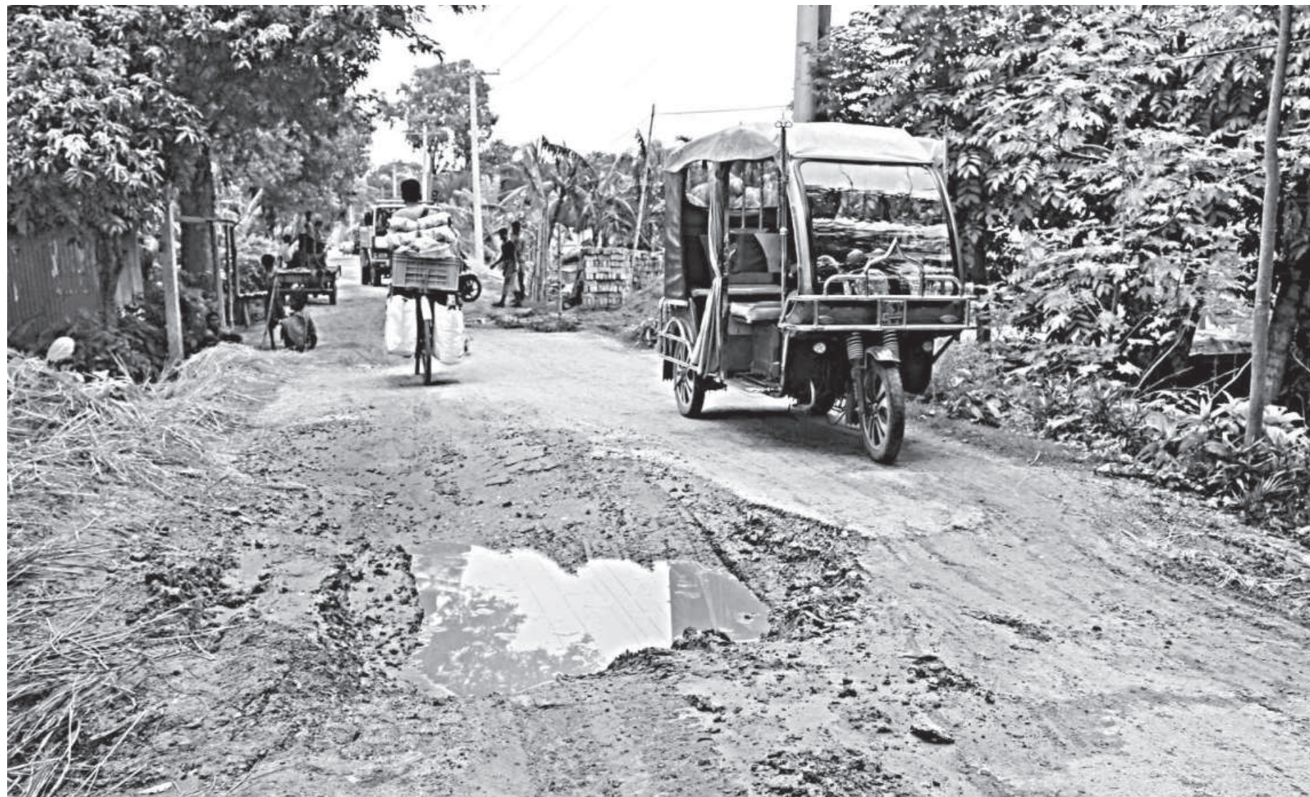
A scene of the Gandimara-Old Belgachhi Bazar road in Rajbari.
