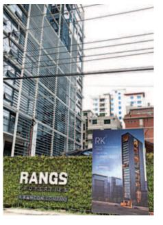
The new version features geotextile bags. These little bags or pockets work as a container for a compound mixture, where plants can grow. The fence is densely aligned with many of these bags making it a green fence. This version is sustainable and is 40 percent less expensive compared to the original version.
