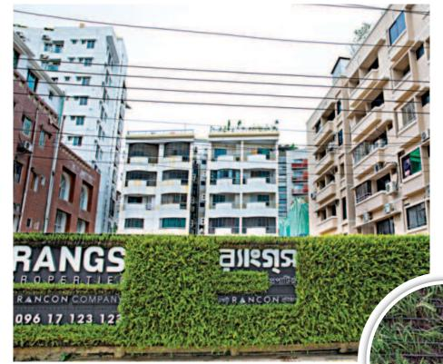
The new version features geotextile bags. These little bags or pockets work as a container for a compound mixture, where plants can grow. The fence is densely aligned with many of these bags making it a green fence. This version is sustainable and is 40 percent less expensive compared to the original version.
