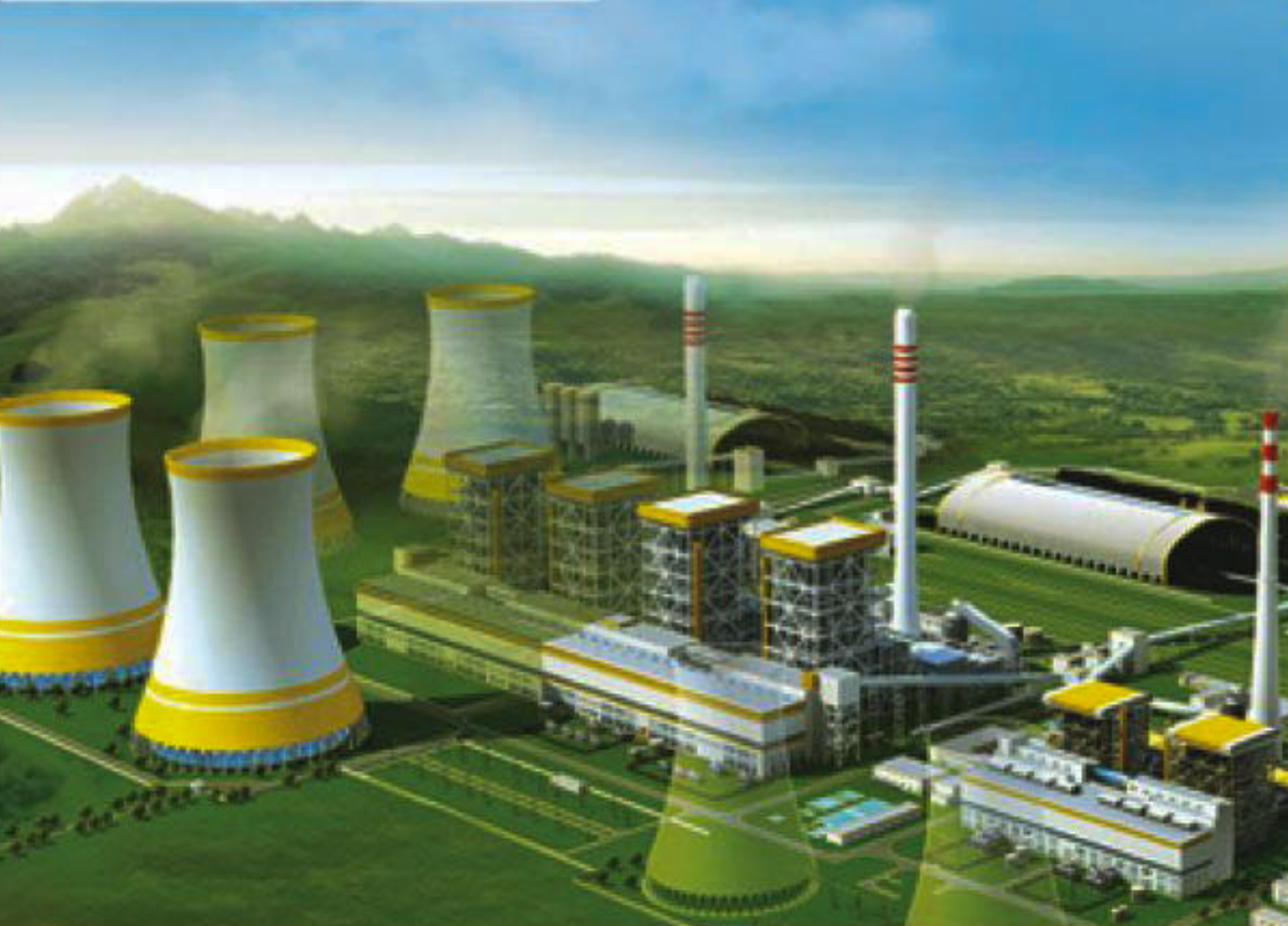
Matarbari Power Plant
