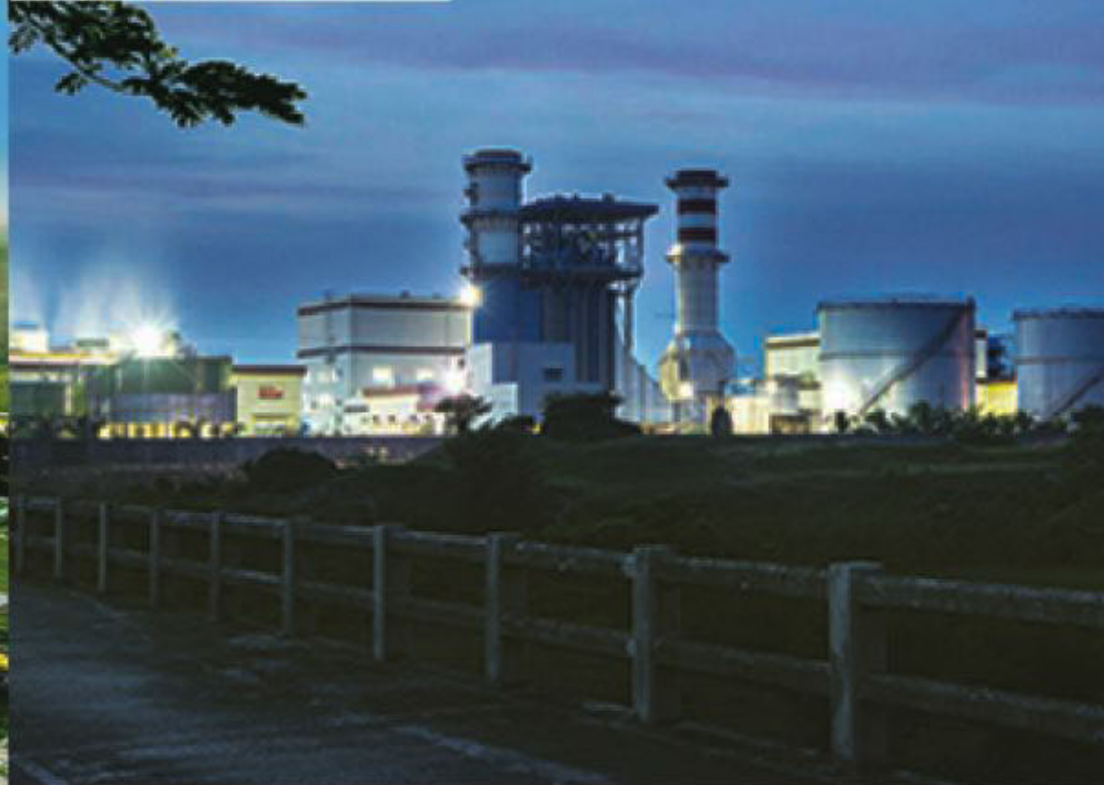
Sirajgonj Power Plant
