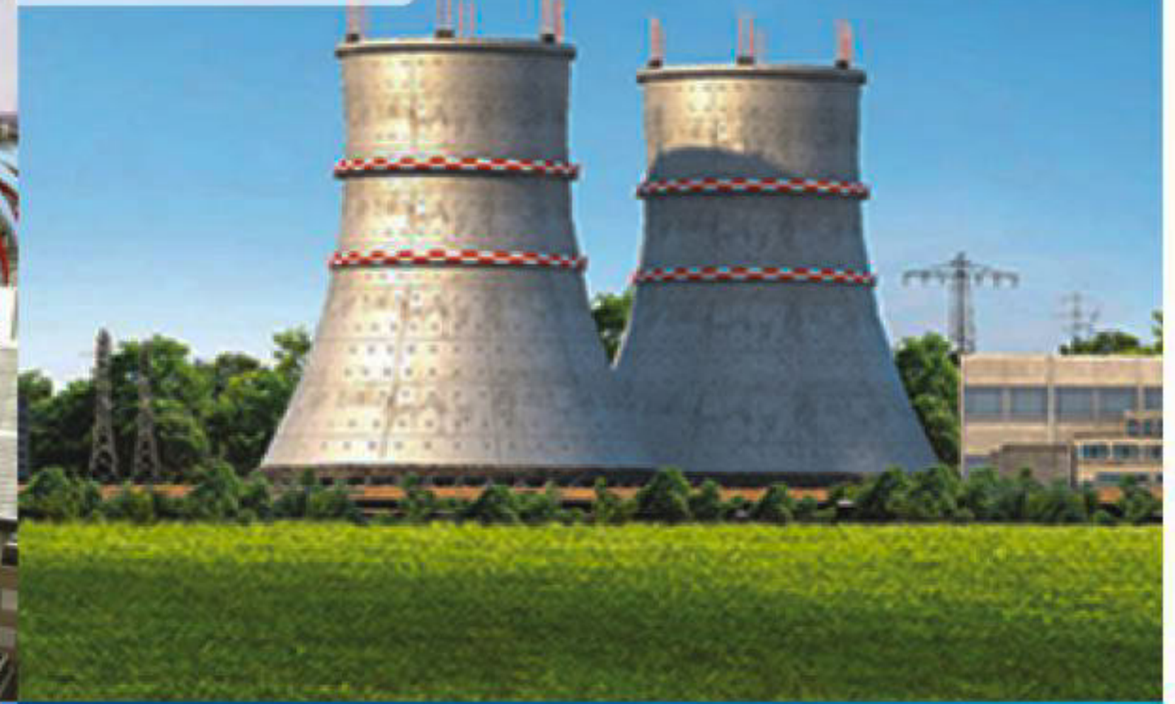
Rooppur Nuclear Power Plant
