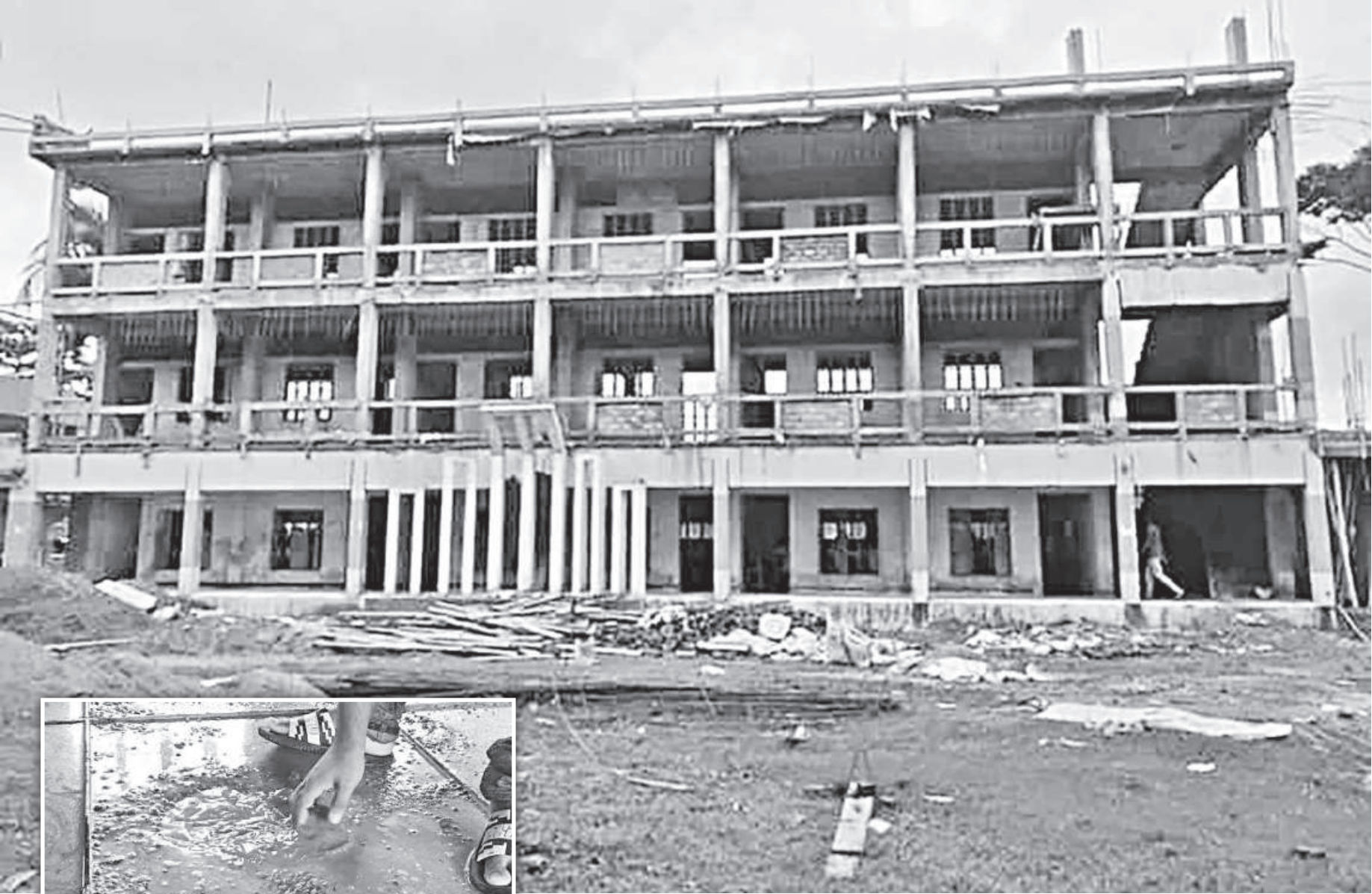
Bhukshimoil School and College in Moulvibazar's Kulaura upazila. Inset, the floor of the institution building's extended part loosens after only a little effort with bare hands as very low quality materials were allegedly used for the work.
