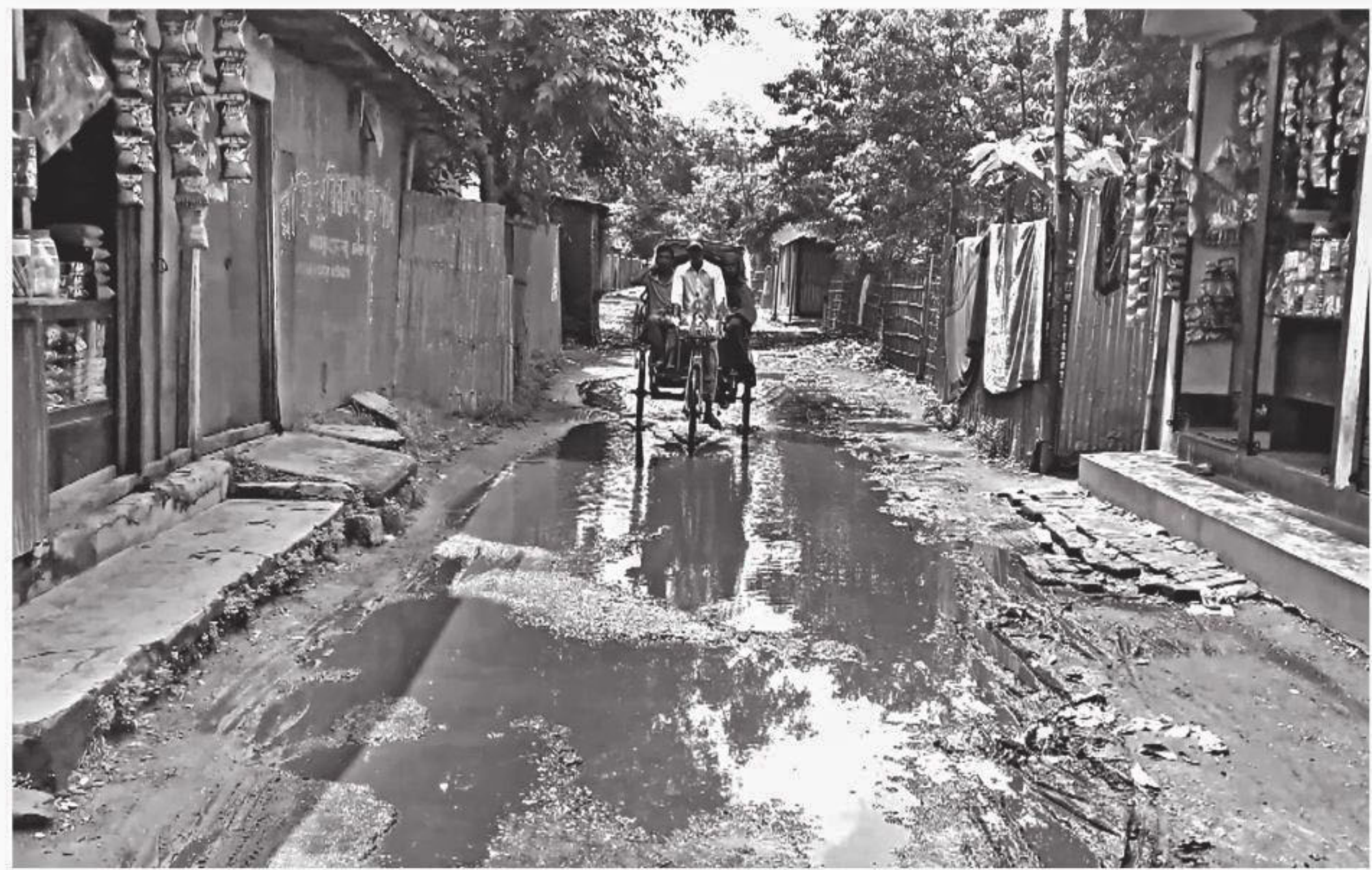
Station Road in Lalmonirhat town remains in awful state for years, causing immense sufferings to locals.
