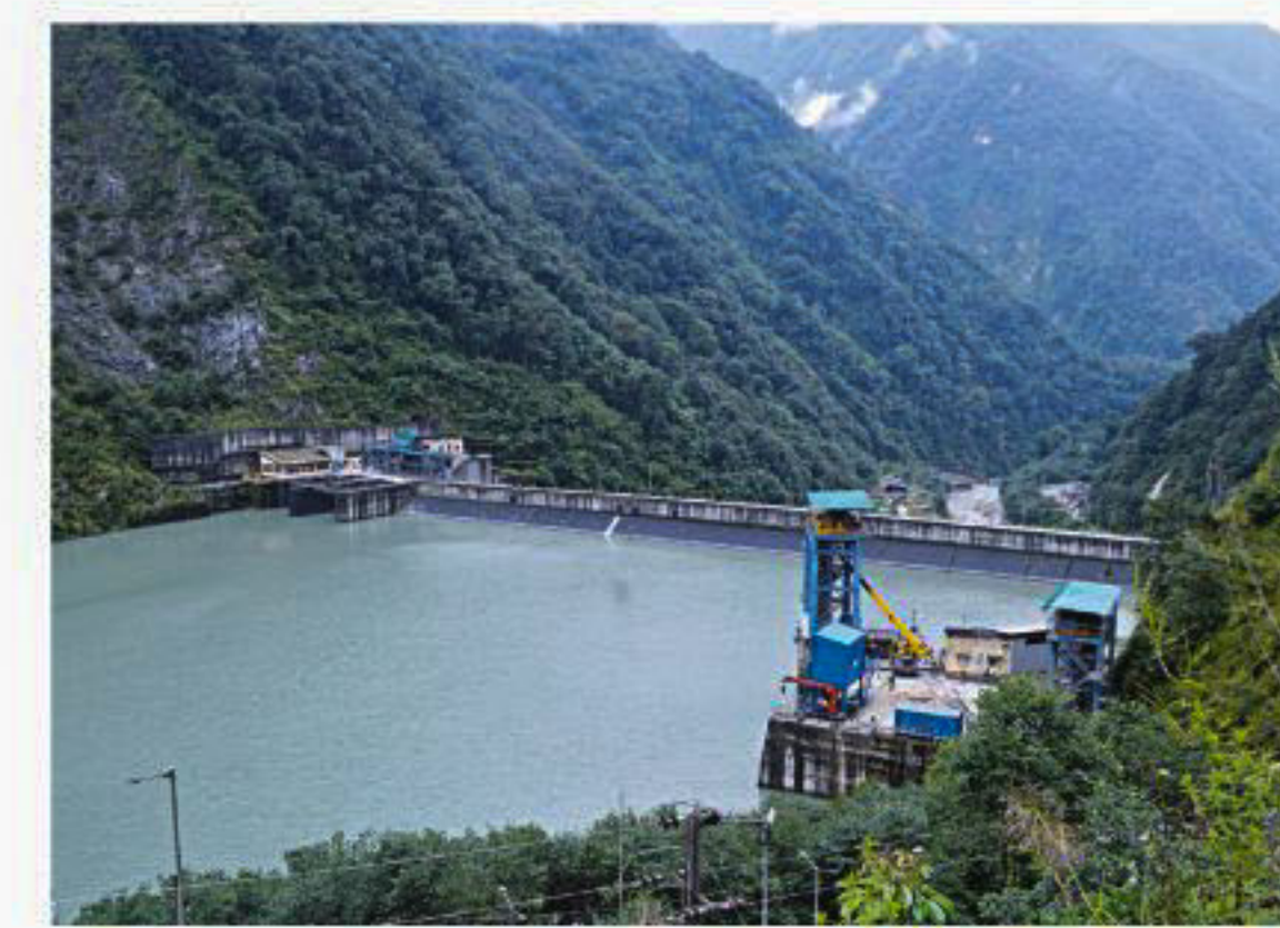
The 1200 MW Chungthang Hydropower plant
