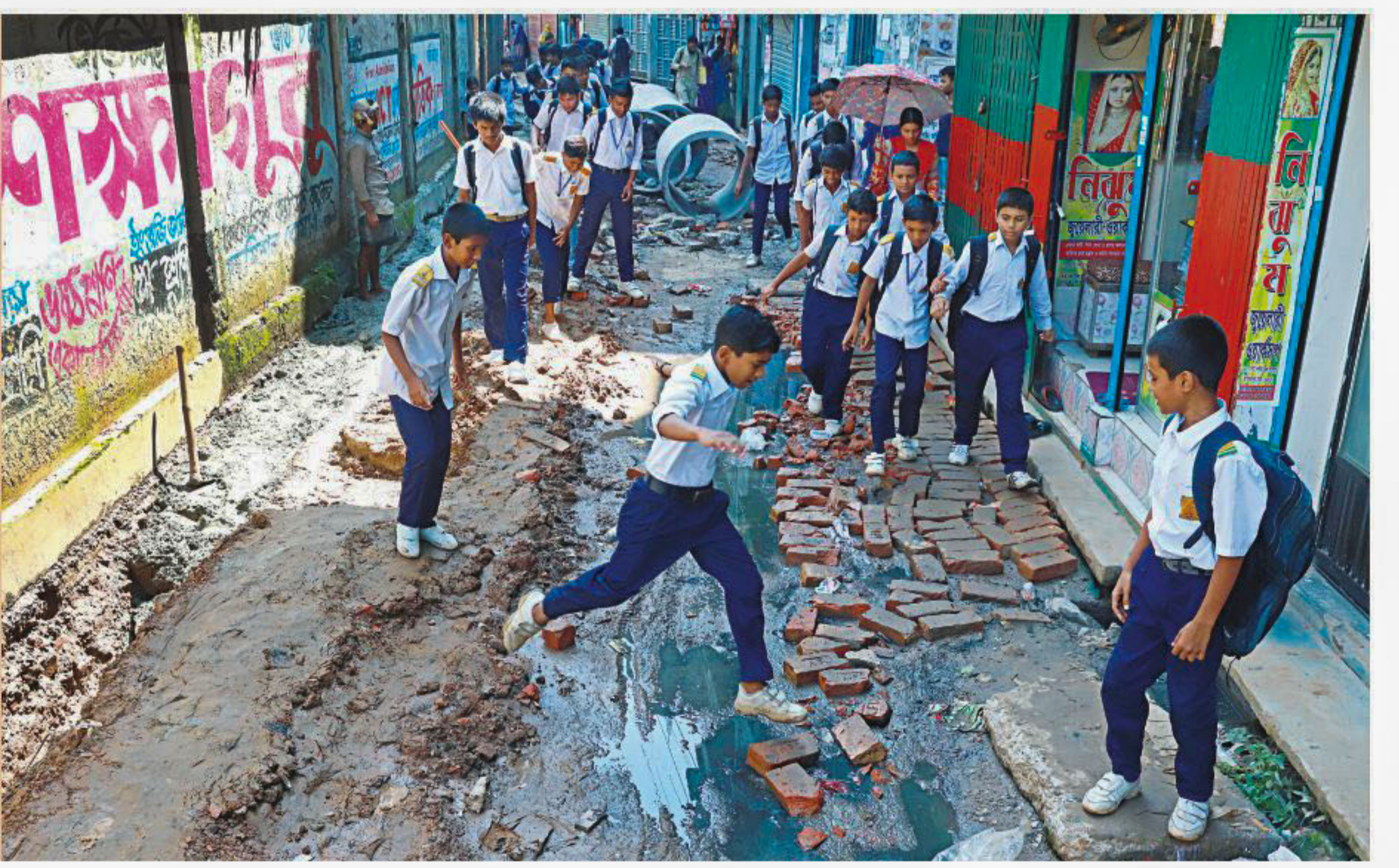
A schoolboy jumps to cross a poorly filled trench dug up by Dhaka South City Corporation in Azimpur area of the capital. Locals said the street has been in this condition since the DSCC started installing sewer lines about a month and half ago. The photo was taken on Wednesday. PHOTO: AMRAN HOSSAIN
